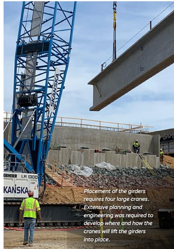
*Placement of the girders requires four large cranes. Extensive planning and engineering was required to develop where and how the cranes will lift the girders into place.*
