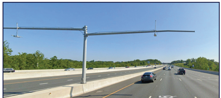
Reconstructed roadway - four general purpose lanes in each direction with two northbound ETL
