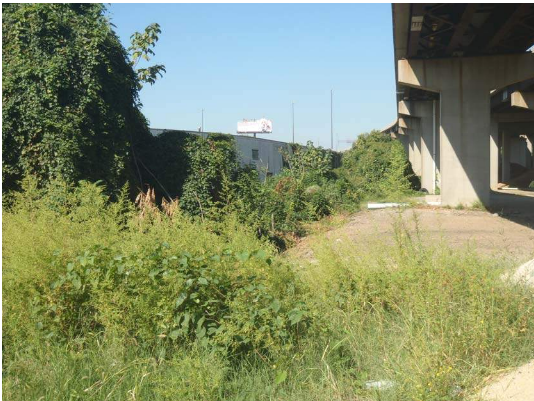
Figure D-6. View west towards north/east side of Howard Uniform Company Building, below east side of I-95 .
