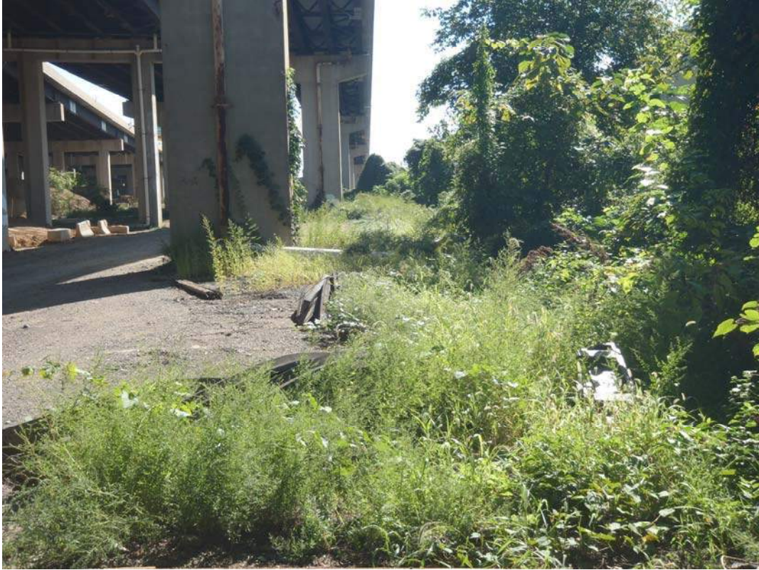
Figure D-5. View east from north side of Howard Uniform Company Building below east side of I-95.
