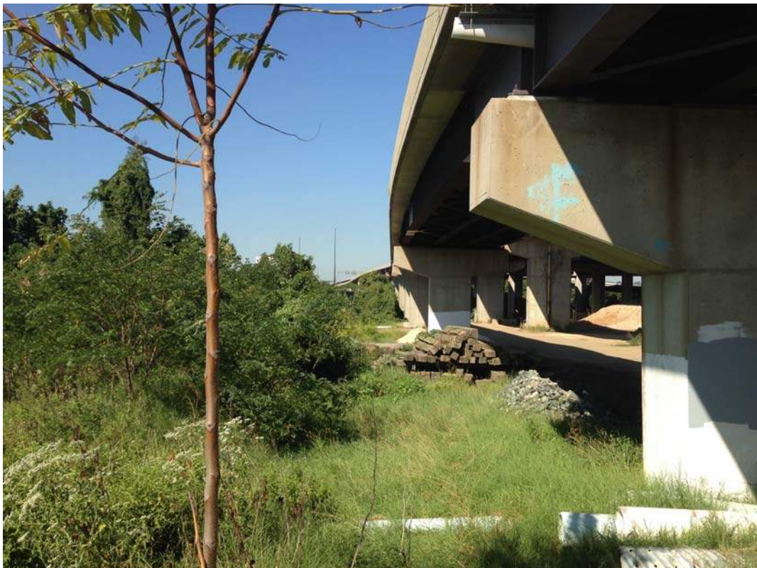
Figure D-10. View east towards the Middle Branch from the east side of the MTA light rail line
