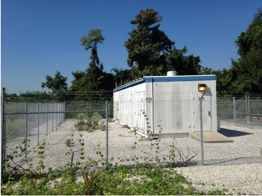
Figure D-11. View south of MTA utility building within architectural APE.
