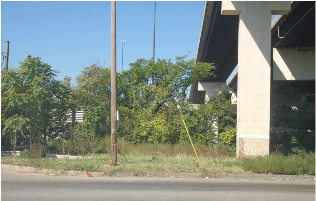
Figure D-4. View west between I-95 and South Monroe Street from Howard Uniform Company Parking Lot (1915 Annapolis Road).
