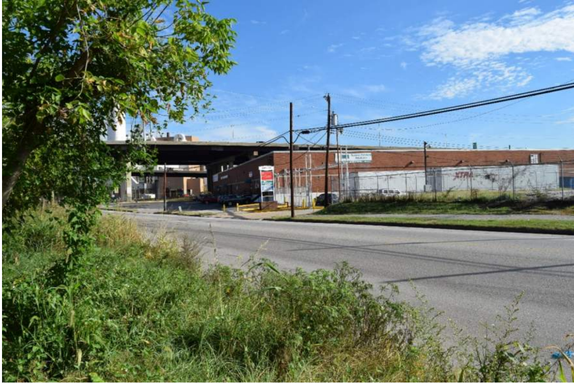
South and west elevations of the Warehouse and Distribution Facility at 1915-1921 Annapolis Road, facing north. Image file: Warehouse and Distribution Center_2017-10-10_01.TIF
