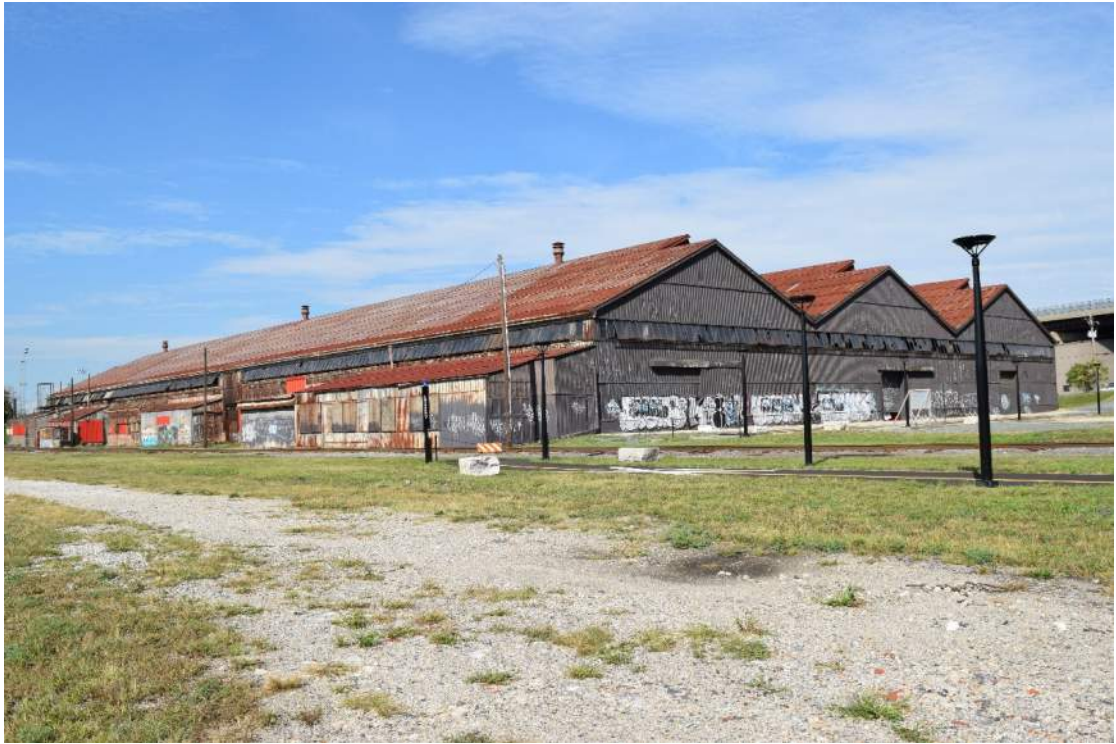
South and east elevations of Lyon, Conklin & Company, facing northwest. Image file: B-1055_2017-10-10_02.TIF
