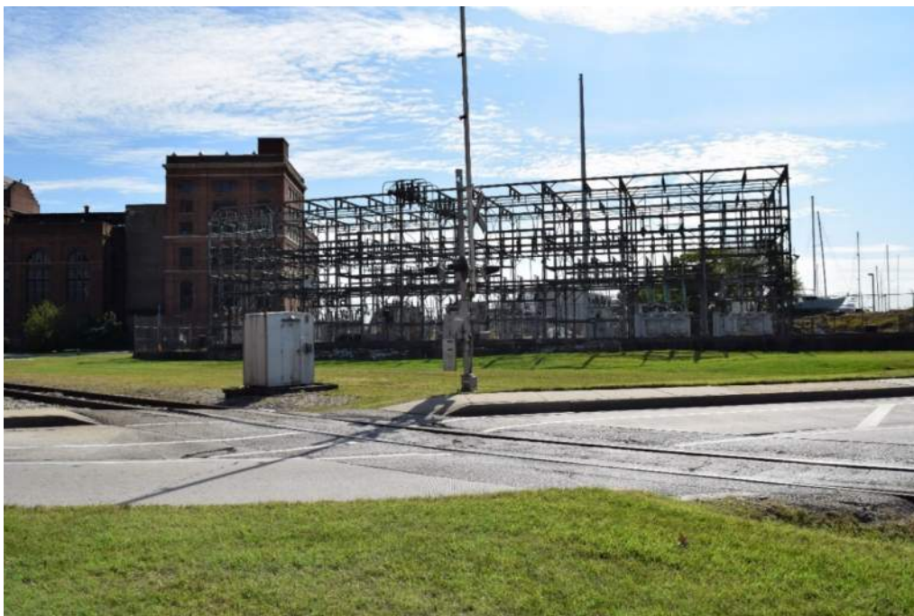
North elevation of Gould Street Generating Station switch house and electrical substation, facing south. Image file: B-5309_2017-10-10_02.TIF
