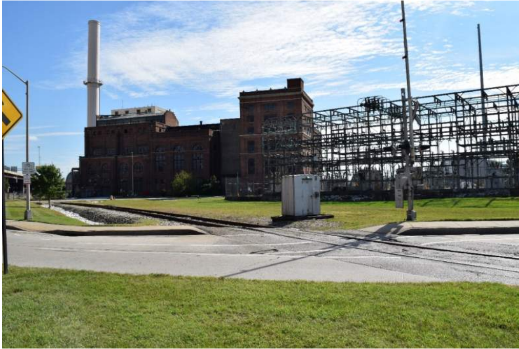
North elevation of Gould Street Generating Station, facing south, showing 1905 coal preparation plant (left) and 1930 switch house (right). Image file: B-5309_2017-10-10_01.TIF
