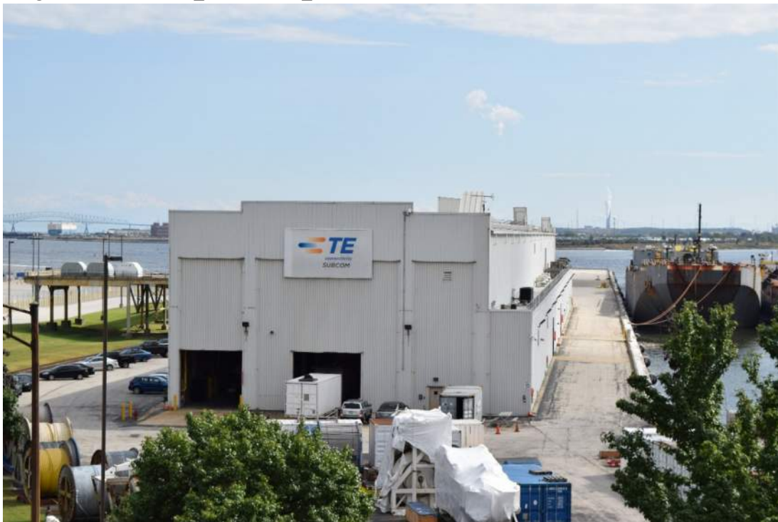
North elevation of the northern warehouse at 1001 E. McComas Street, facing south towards the water. Image file: Warehouse_10-10-2017_02.TIF
