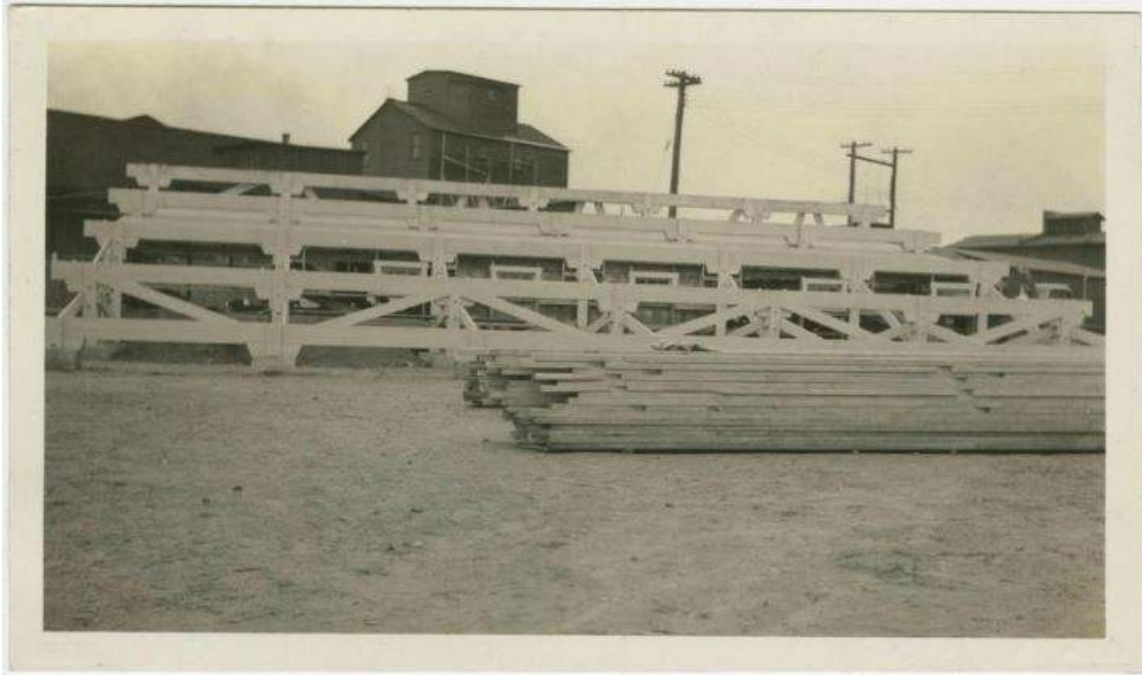
Figure 1. Works Progress Administration, Grandstand at Swann Park, April 21, 1936 (Source: University of Maryland Libraries Digital Collections)
