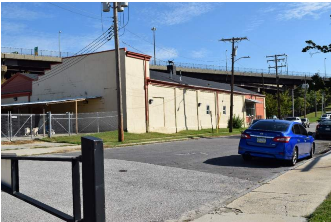
South and west elevations of warehouse at 200 West McComas Street, facing northeast. Image file: Storage Warehouse_2017-10-10_02.TIF
