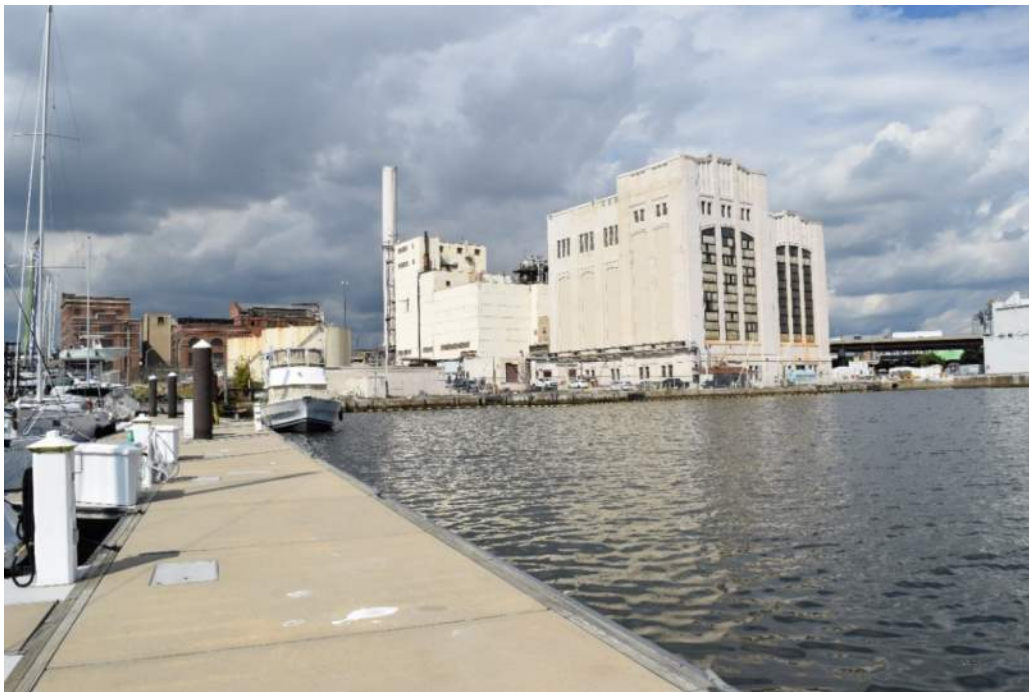
South and west elevation of Gould Street Generating Station Steam Generating Plant, facing northeast. Image file: B-5309_2017-10-10_04.TIF
