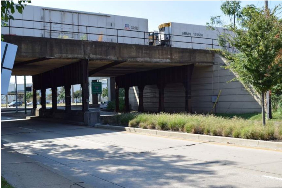
Northern elevation of Baltimore and Ohio Rail Bridge over Key Highway, facing southwest. Image file: B-5311_2017-10-10_01.TIF
