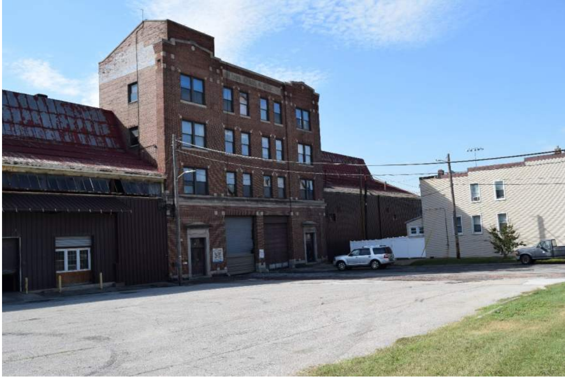
North elevation of Lyon, Conklin & Company, facing southwest. Image file: B-1055_2017-10-10_01.TIF
