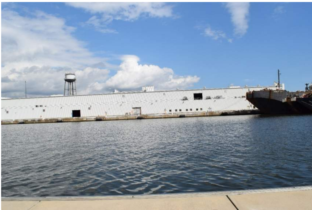
Middle west elevation of the northern warehouse at 1001 E. McComas Street, facing east. Image file: Warehouse_2017-10-10_04.TIF
