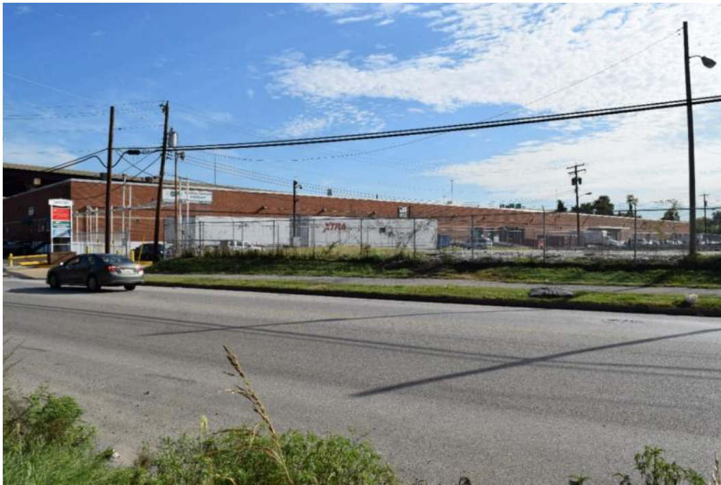
South and partial west elevations of the Warehouse and Distribution Facility at 1915-1921 Annapolis Road, facing northeast. Image file: Warehouse and Distribution Center_2017-10-10_02.TIF
