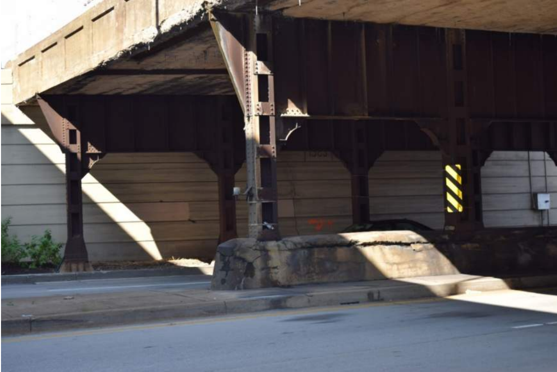
Detail of bent on Baltimore and Ohio Rail Bridge over Key Highway, facing west. Image file: B-5311_2017-10-10_03.TIF
