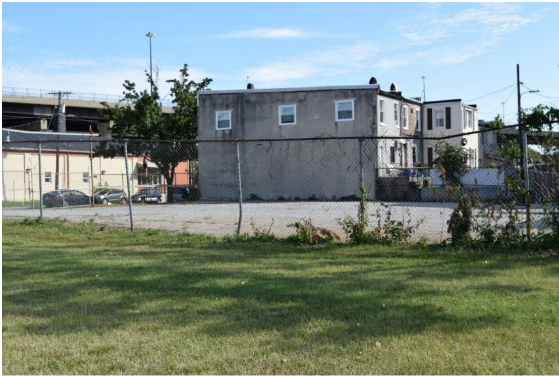
West elevation of 201-213 W. McComas Street, facing east. Image file: B-5310_2017-10-10_02.TIF
