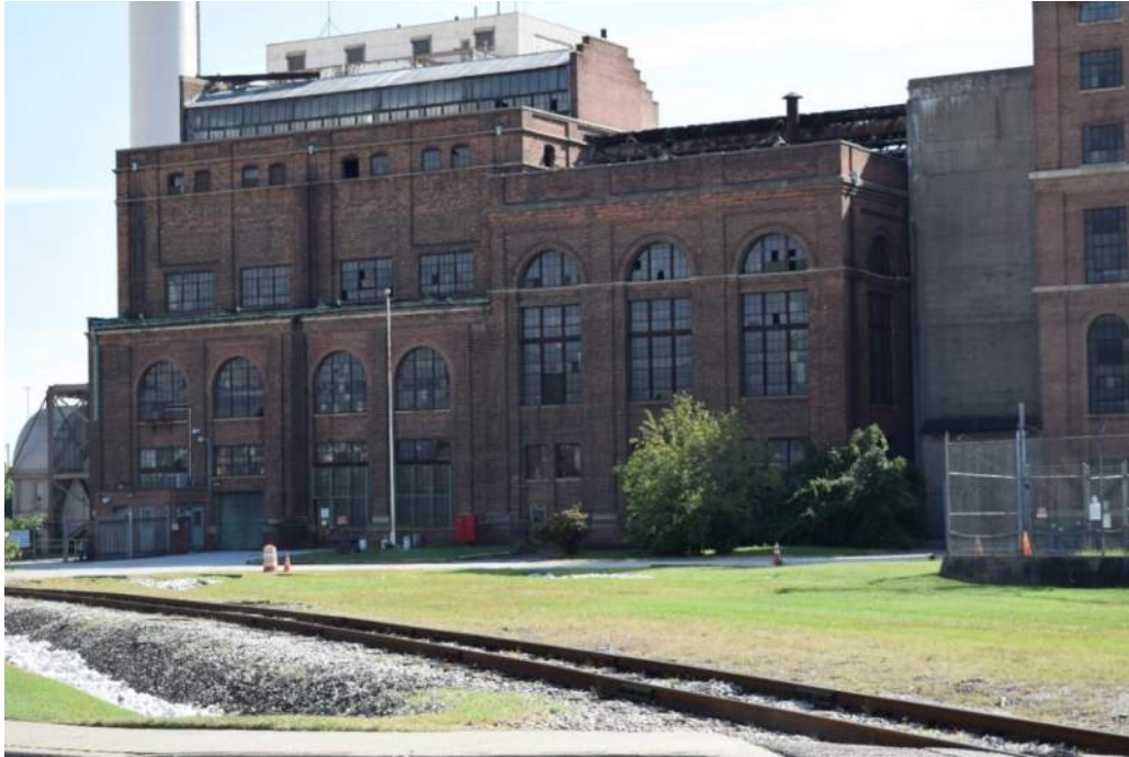
Close-up of Gould Street Generating Station 1905 structure north elevation, facing south. Image file: B-5309_2017-10-10_03.TIF
