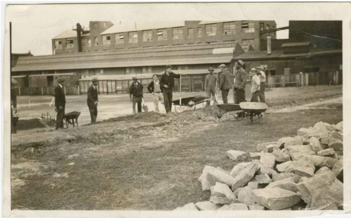
Figure 2. Works Progress Administration, Construction of athletic fields at Swann Park, November 4, 1936 (Source: University of Maryland Libraries Digital Collections).
