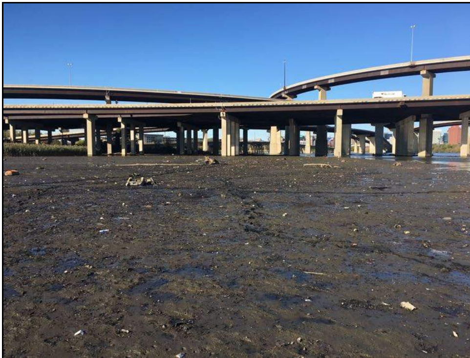
Figure 6. Photograph Looking North, Western Side of the Survey Area (Low Tide).
