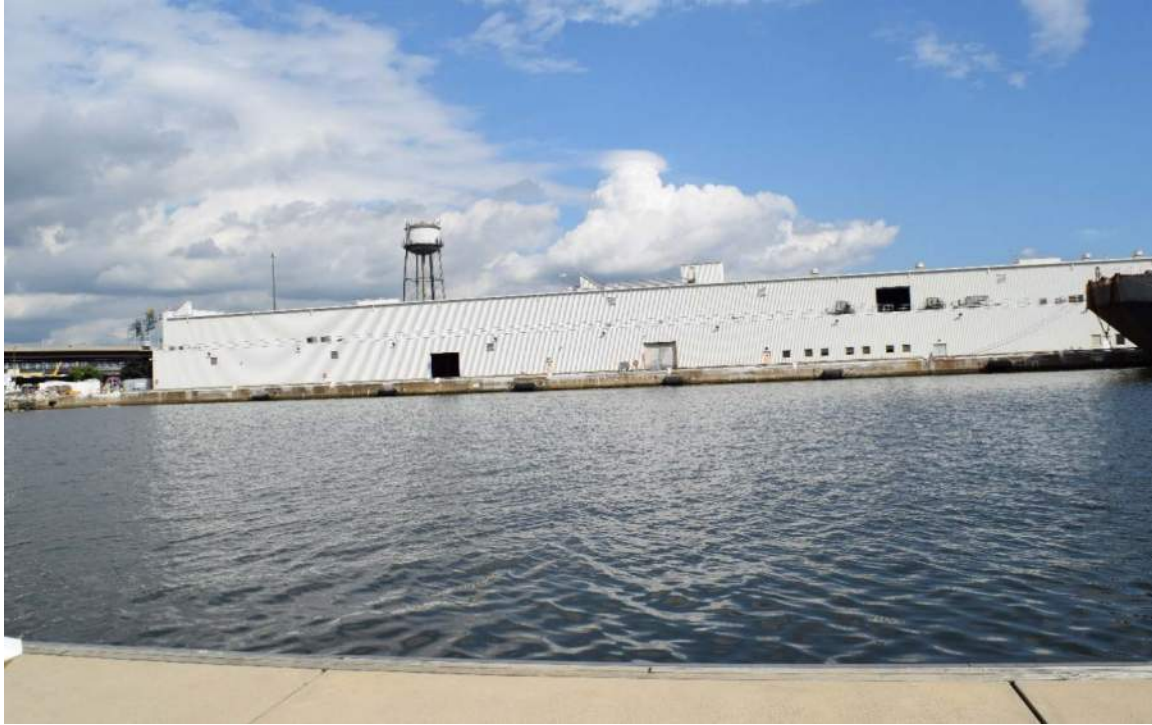
Western elevation of the northern warehouse at 1001 E. McComas Street, facing northeast. Image file: Warehouse_2017-10-10_03.TIF
