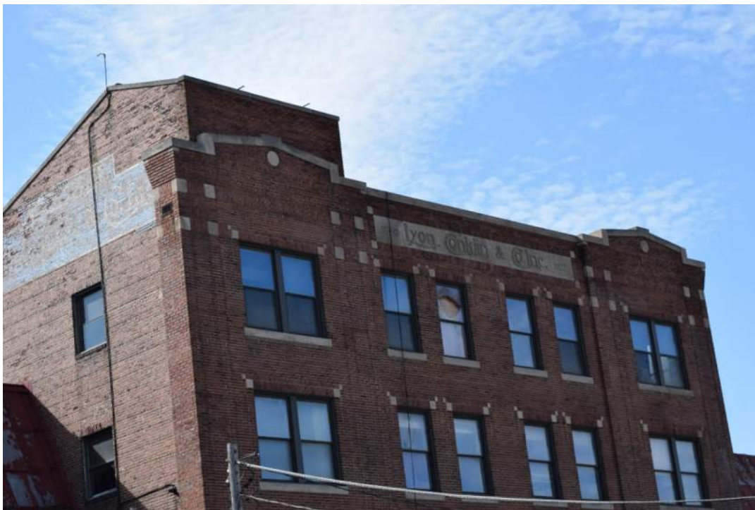
North elevation of Lyon, Conklin & Co. building showing the brick façade and “Lyon, Conklin, & Co.” sign, facing southwest. Image file: B-1055_2017-10-10_04.TIF
