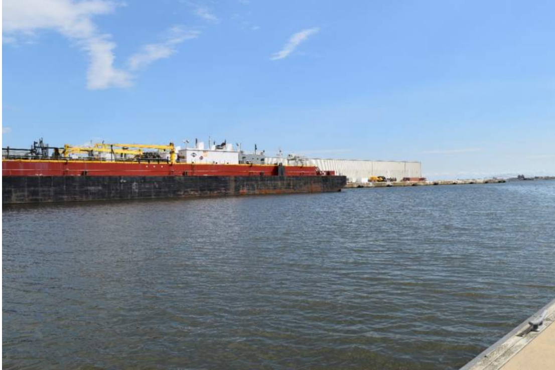
Western elevation of the south warehouse at 1001 E. McComas Street, facing southeast. Image file: Warehouse_2017-10-10_01.TIF
