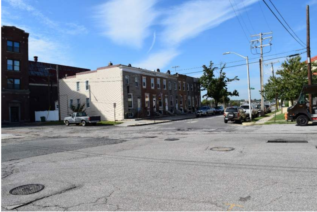
North and east elevations of 201-213 W. McComas Street, facing southwest. Image file: B-5310_2017-10-10_01.TIF
