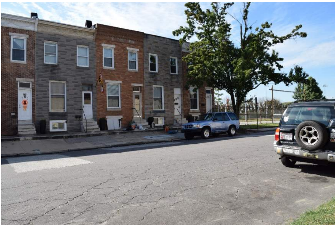
North elevation of 207-213 W. McComas Street, facing southwest. Image file: B-5310_2017-10-10_04.TIF
