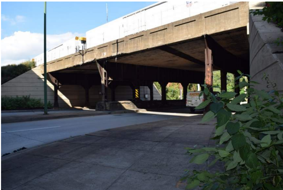
Southern elevation of Baltimore and Ohio Rail Bridge over Key Highway, facing northwest. Image file: B-5311_2017-10-10_02.TIF
