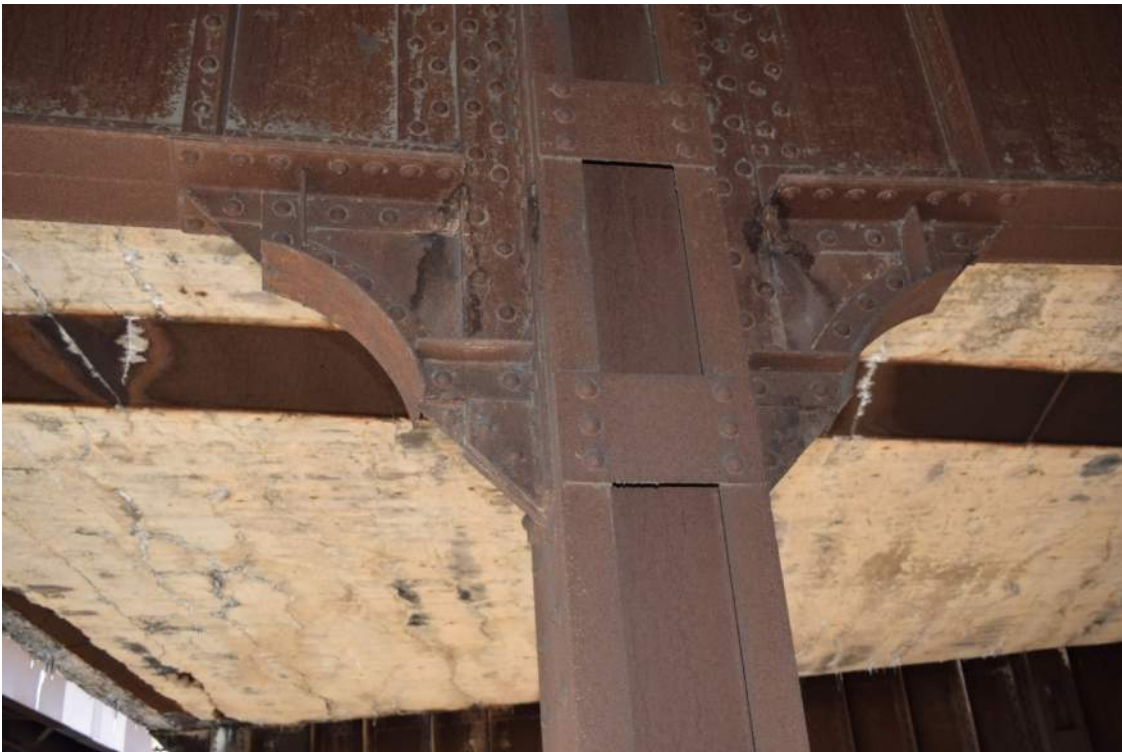
Pier detail of Baltimore and Ohio Rail Bridge over Key Highway, facing west. Image file: B-5311_2017-10-10_04.TIF
