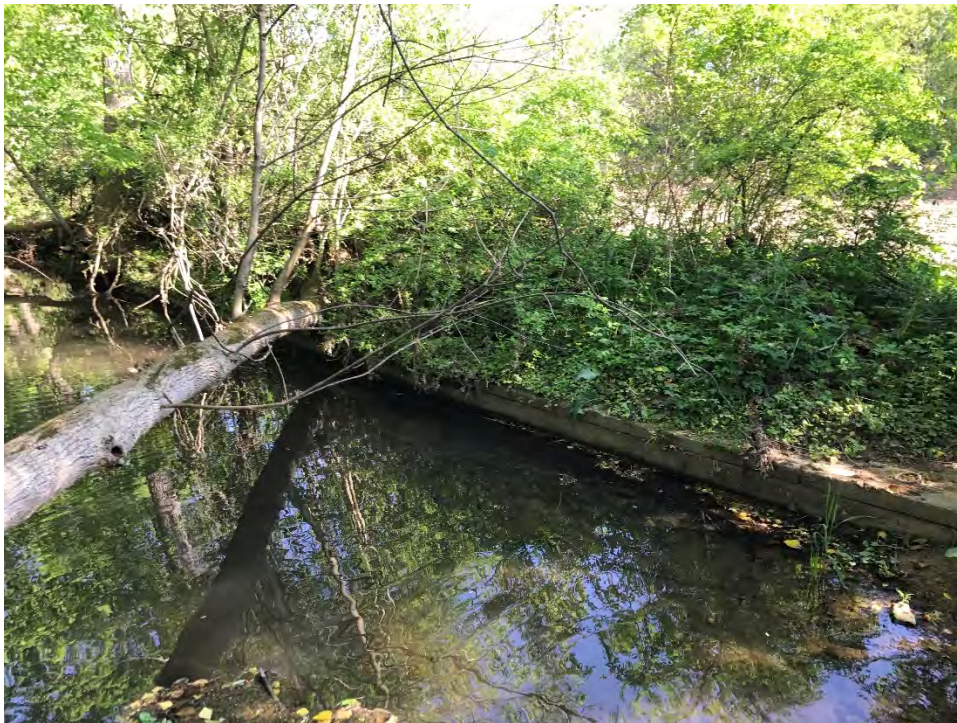
Figure 18: Concrete wall in channel upstream of concrete dam in Middle Jones
