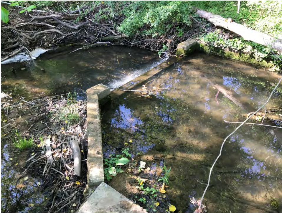
Figure 19: Concrete dam in Middle Jones
