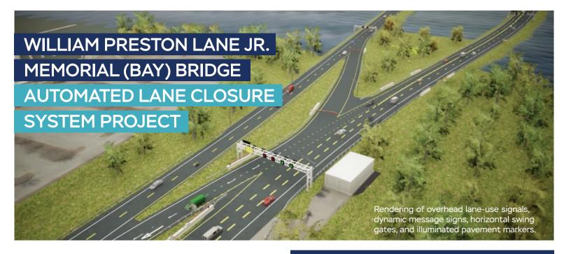
The Bay Bridge automated lane closure system (ALCS) is a project constructed for opening and closing lanes for two-way traffic operations on the bridge. Since two-way operations were implemented, lane closures have been done manually. The ALCS will enhance the current cone and barrel system by allowing remote implementation and discontinuation of two-way traffic on the Bay Bridge's Eastern and Western shores.
