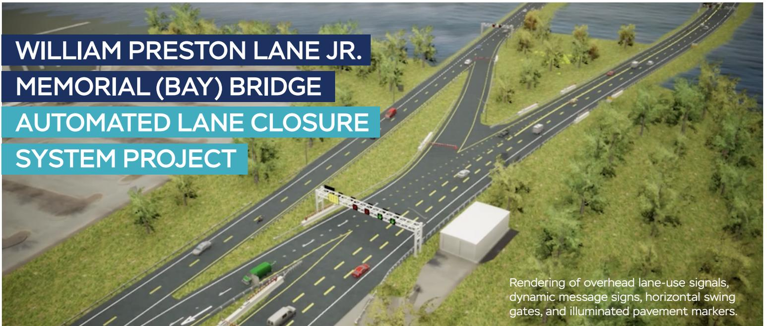
Rendering of overhead lane-use signals, dynamic message signs, horizontal swing gates, and illuminated pavement markers.
