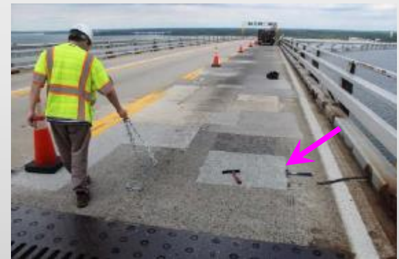
View of WB Right Lane with patching & deterioration
