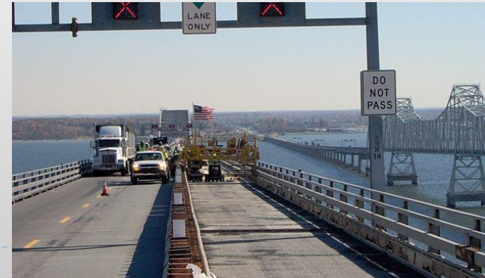
View of WB Left Lane emergency replacement in 2004
