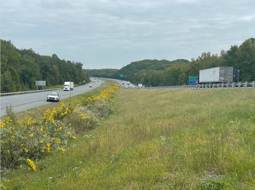
I-95 Bioswale Plantings
