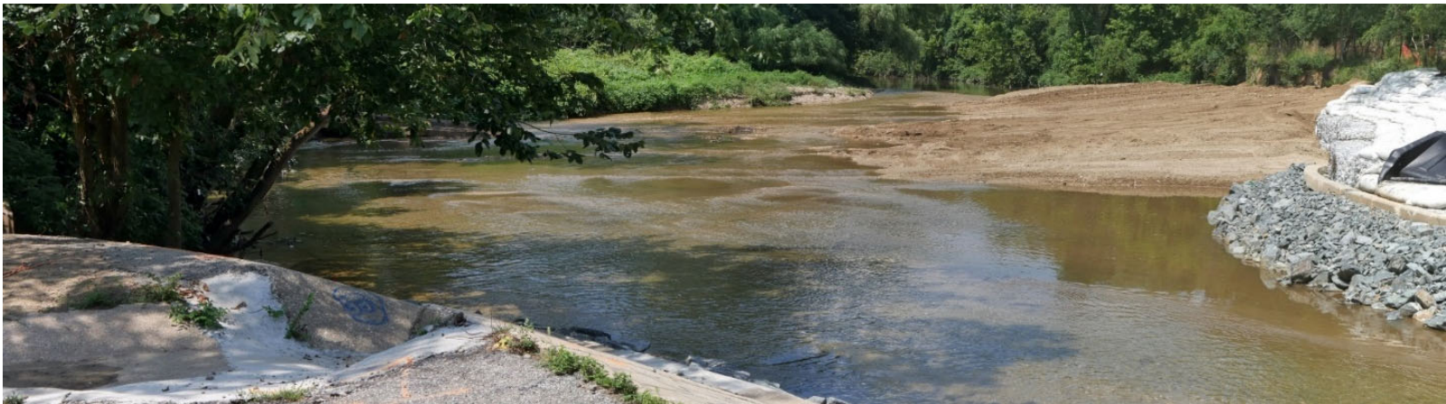
Stream Sediment Bar Grading
