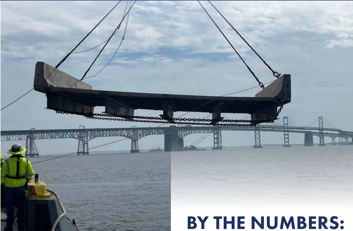
Crews moving precast deck panels into place.
