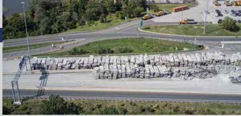
Concrete removed from former Key Bridge.
