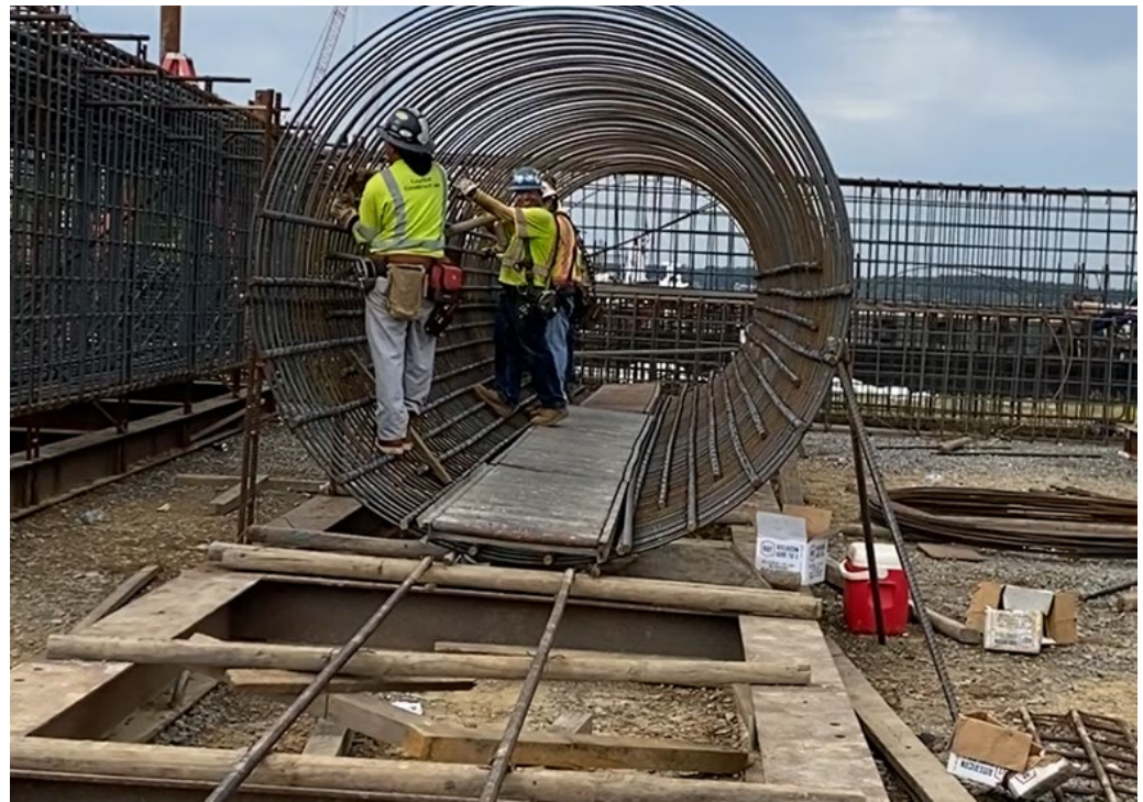
D.T. Read Steel Company, Inc. (DBE Subcontracting firm) tying rebar for bridge piers Bridge Replacement Contract
