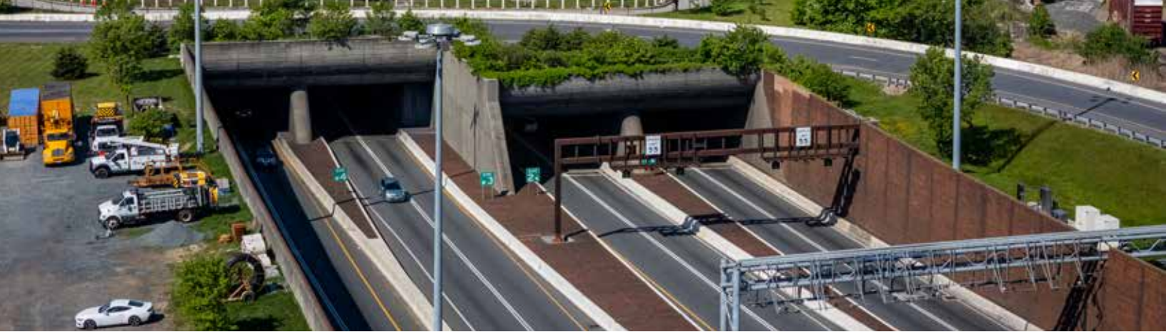
Fort McHenry Tunnel (I-95, I-395)
