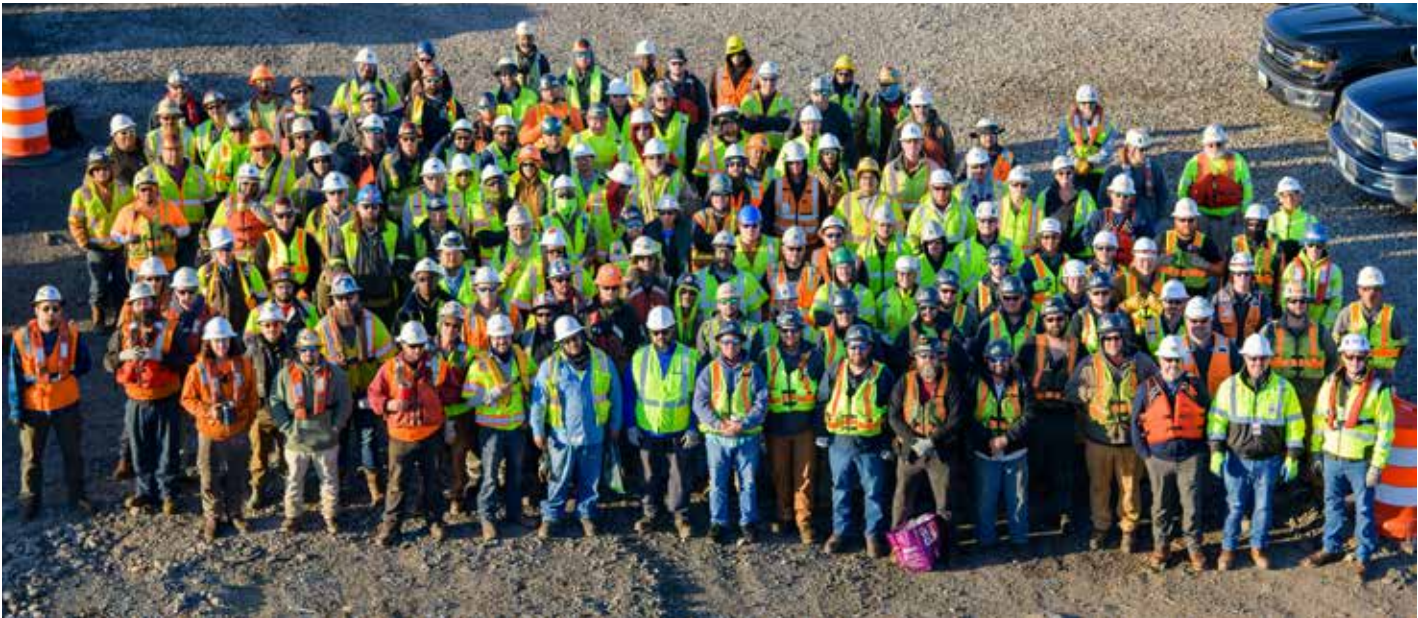
Workers gather for salvage operations of the Francis Scott Key Bridge on the Patapsco River at Sparrows Point, Edgemere, Maryland.
