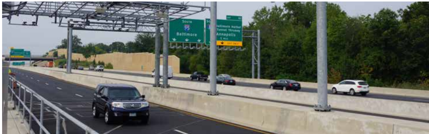
I-95 Express Toll Lanes
