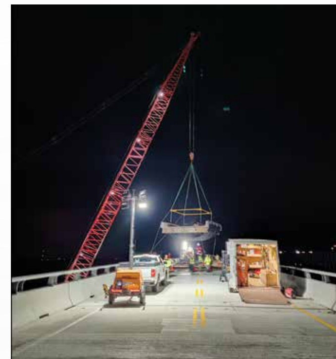
Bay Bridge Eastbound Deck Replacement – March 2025
