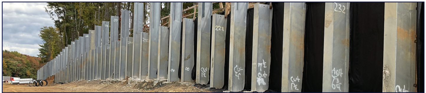
Roadway widening and noise wall currently under construction
