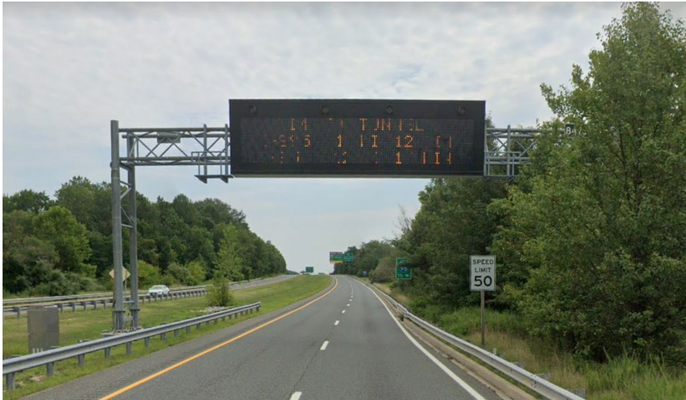
Existing DMS Sign on Southbound MD 43
