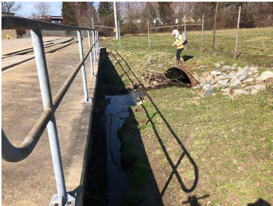
16. WUS 02 FACING NORTHWEST, CULVERT UNDER FIELD
