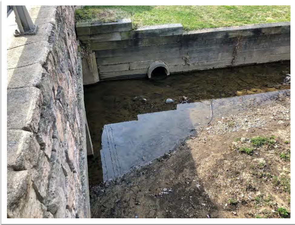
13. WUS 02 FACING WEST, SOUTHERN CULVERT
