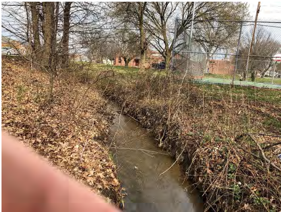
12. WUS 01 FACING NORTHEAST
