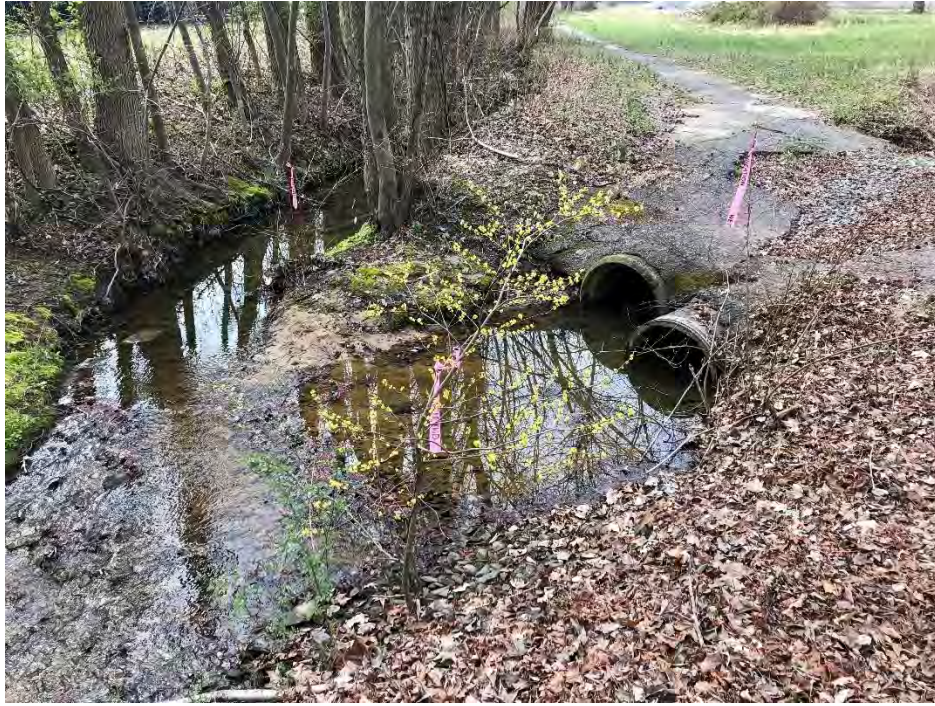
29. WUS 06 FACING SOUTHWEST
