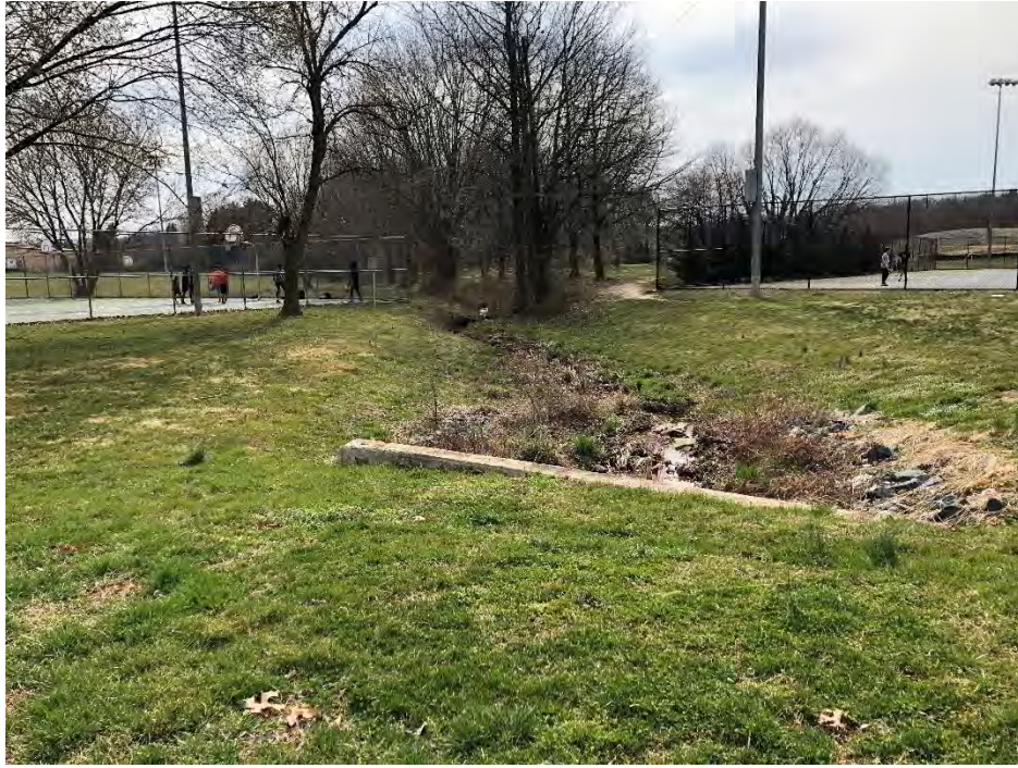
11. WUS 01 FACING SOUTHWEST
