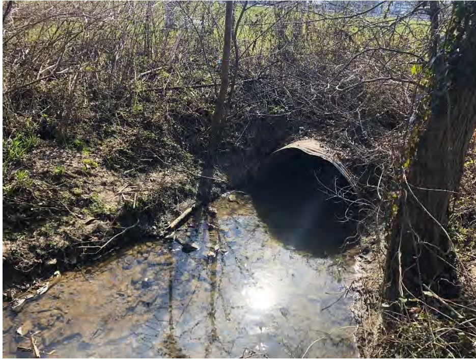
17. WUS 02 FACING SOUTHEAST, END OF CULVERT
