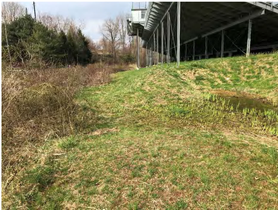
4. WET 02A FACING NORTH
