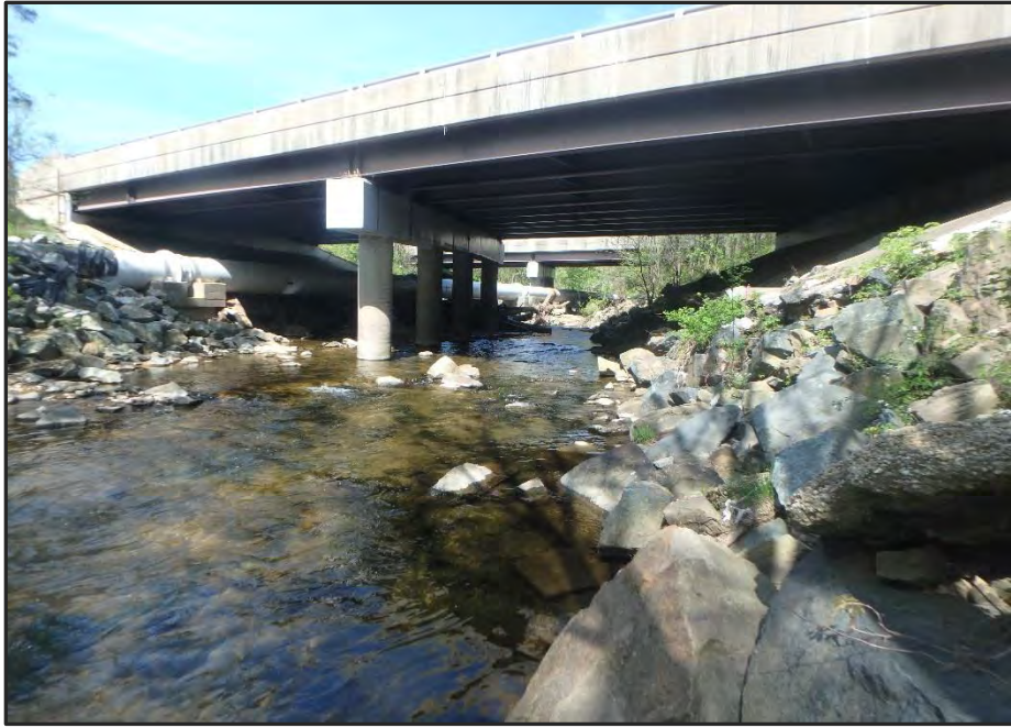
Photo 7: WUS 3D, upstream (Facing Northwest)
