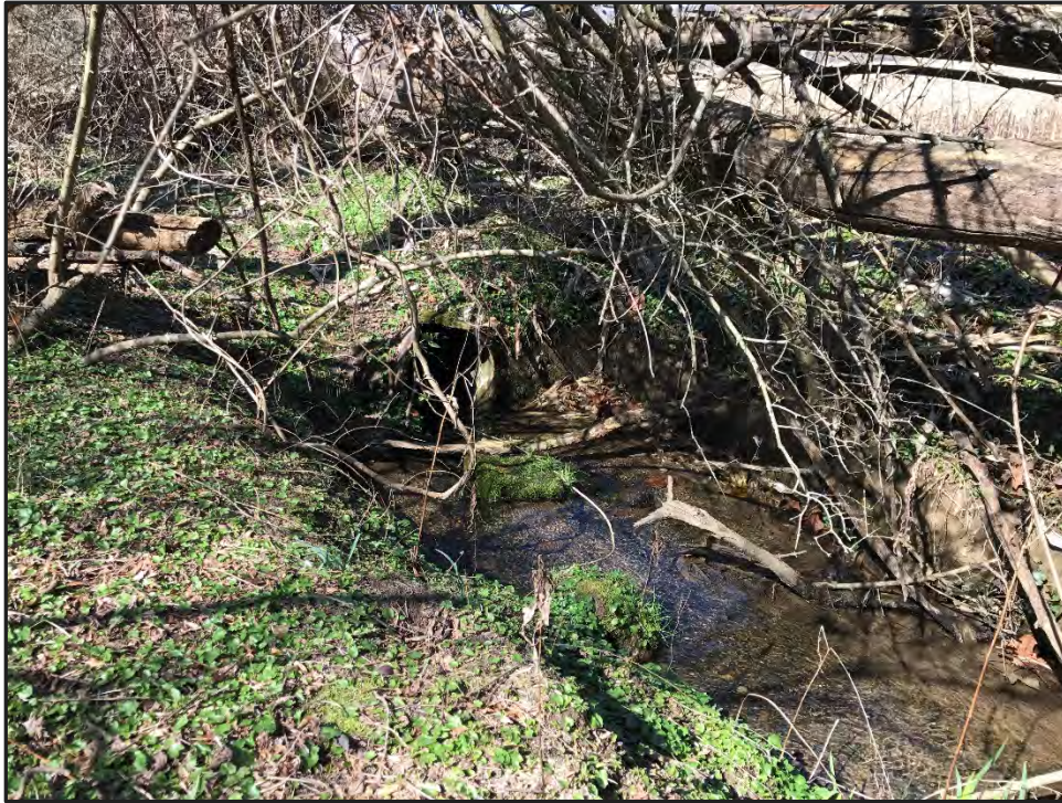
Photo 79: WUS 05 upstream (Facing southwest)
