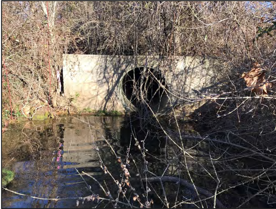
Photo 65: WUS 04 upstream (Facing north)
