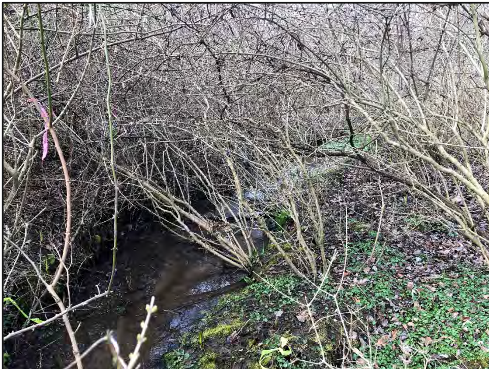
Photo 94: WUS 12 upstream (Facing west)
