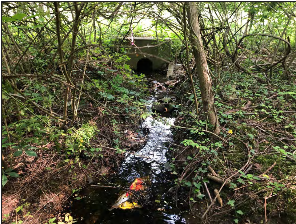
Photo 98: WUS 14 upstream (Facing north)
