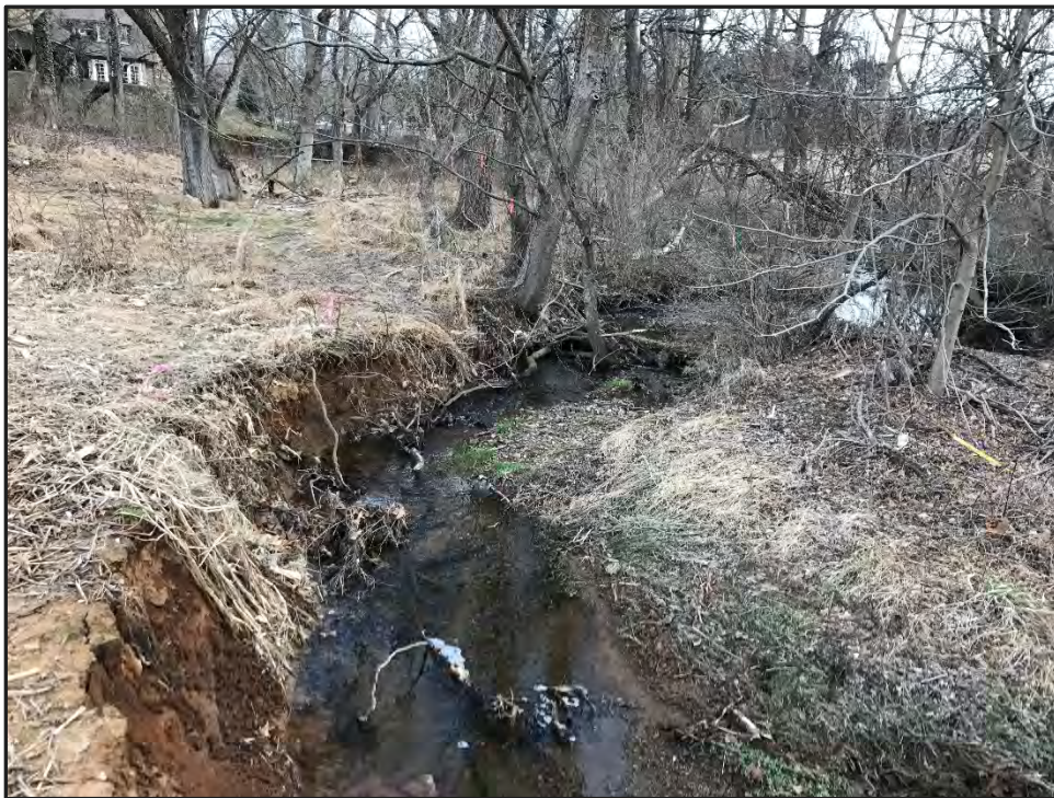
Photo 106: WUS 20 upstream (Facing north)
