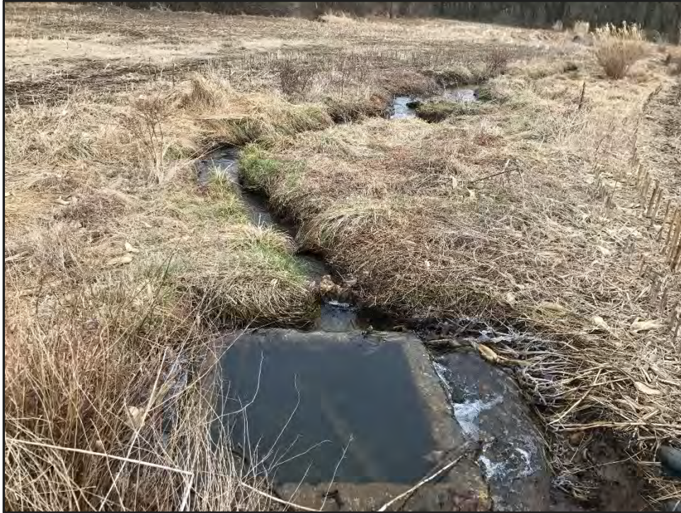
Photo 111: WUS 21 diversion box (Facing south)
