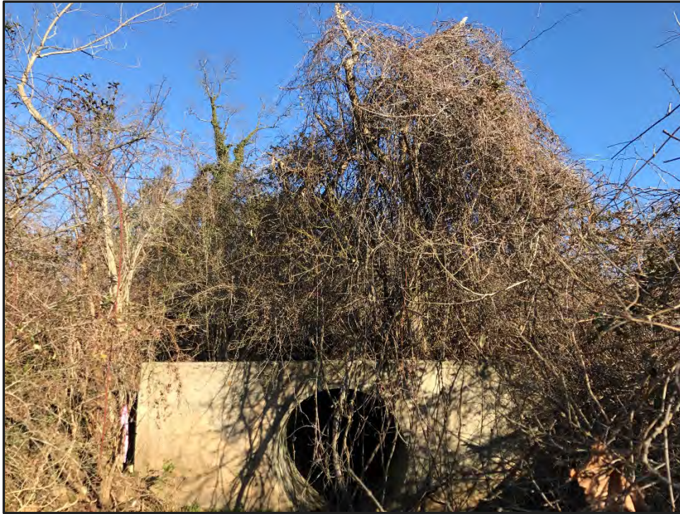
Photo 63: WUS 04 upstream (Facing north)
