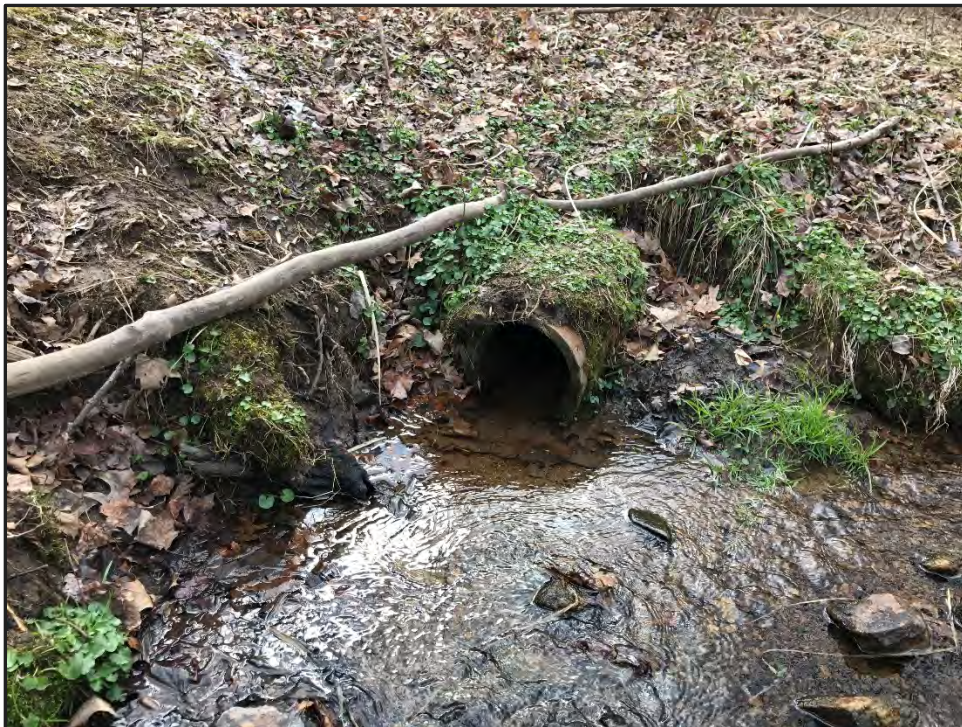
Photo 68: WUS 05 drainage pipe (Facing southwest)
