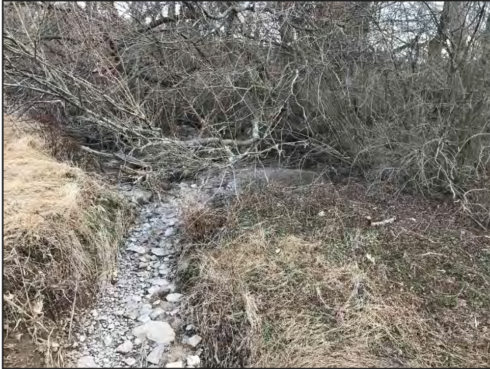
Photo 107: WUS 20 upstream (Facing northeast)
