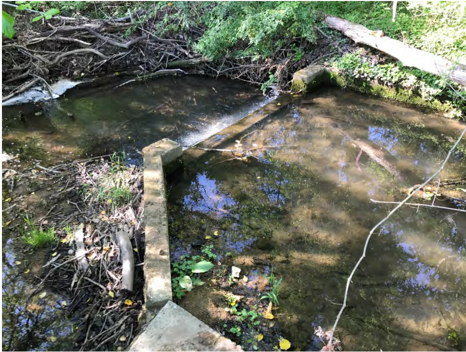
Figure 19: Concrete dam in Middle Jones
