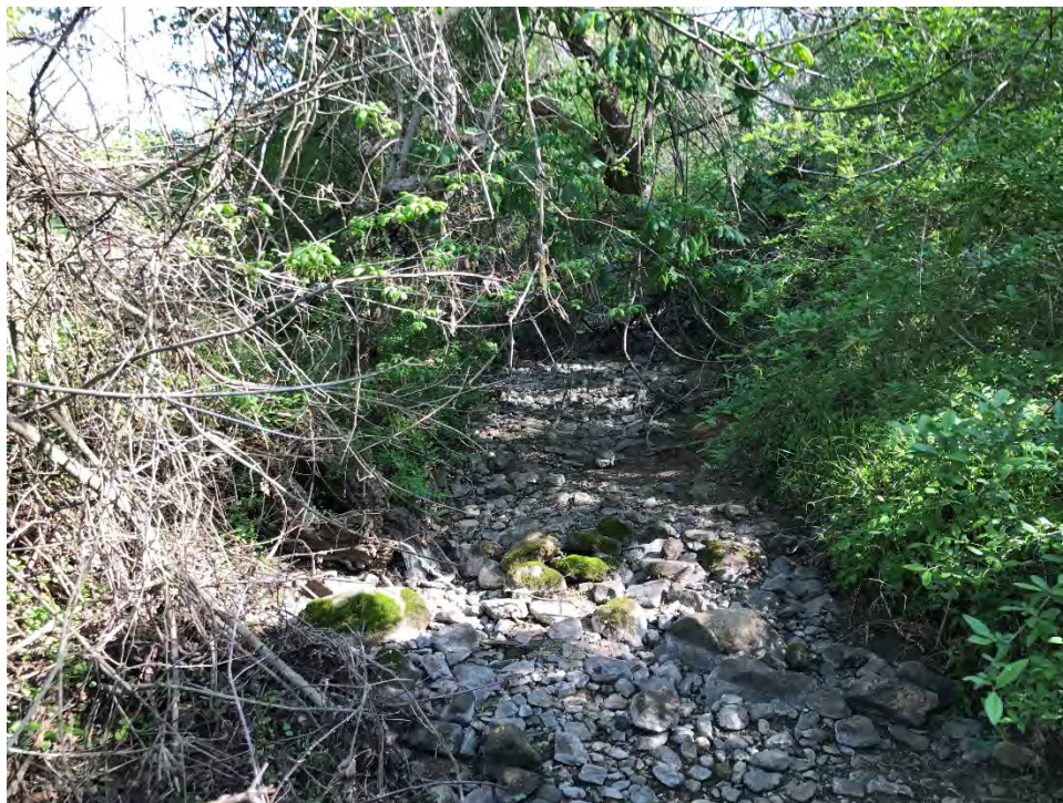
Figure 40: Upstream end of longitudinal profile 6 in Stone House Tributary (looking upstream)
