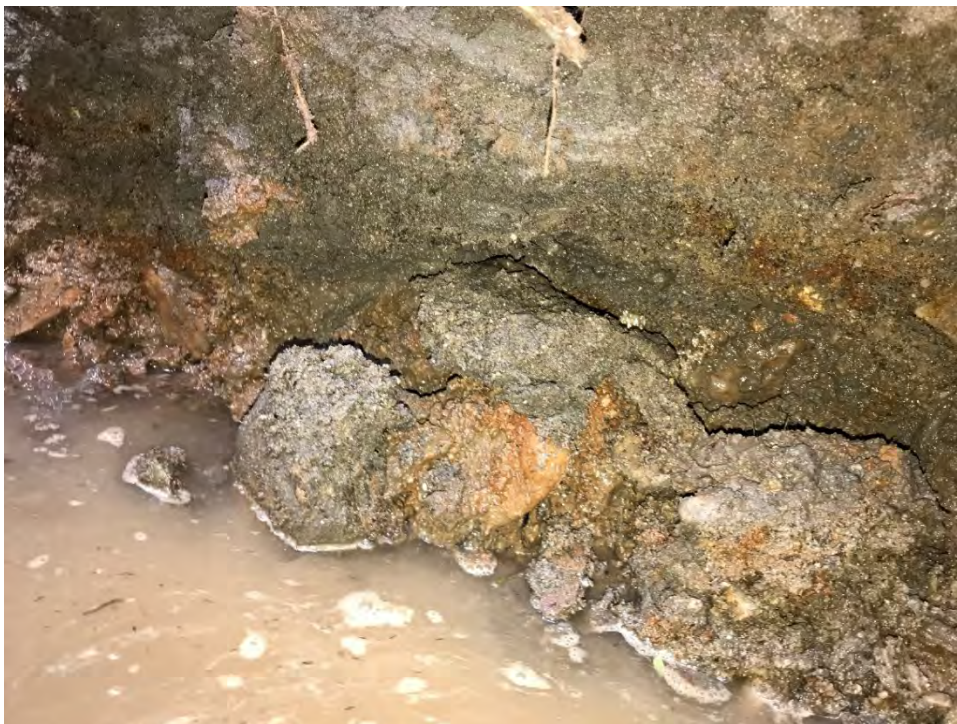
Figure 6: Trench along the main stem of the Jones Falls showing where layers of hydric soil and basal gravel were found
