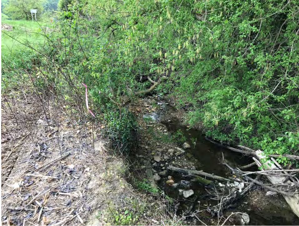
Figure 46: Channel erosion within Intersection Tributary
