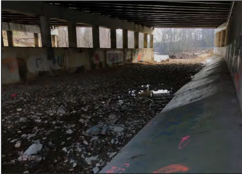
Photo 63: Waters U, downstream (Facing South)
