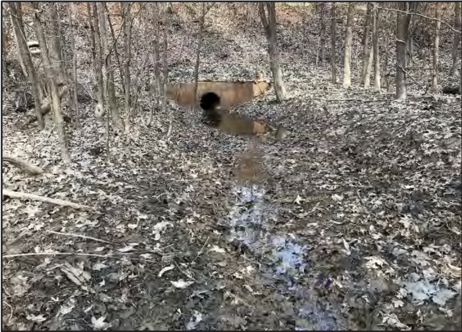
Photo 6: WUS C-3, upstream (Facing North)
