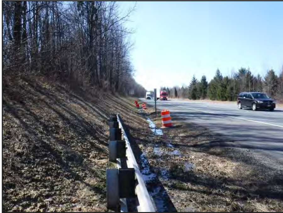
Photo 27: WUS G-16, upstream (Facing West)
