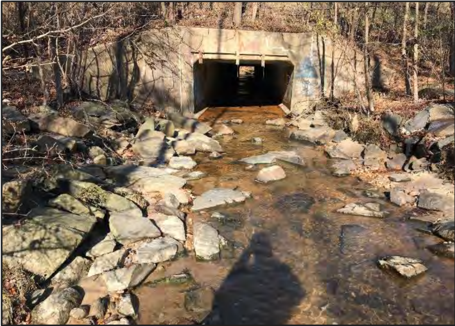
Photo 20: WUS C-10, upstream (Facing North)
