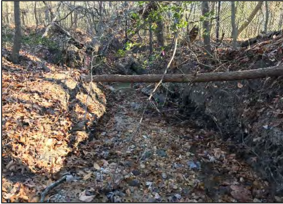
Photo 15: WUS C-8, downstream (Facing Southwest)
