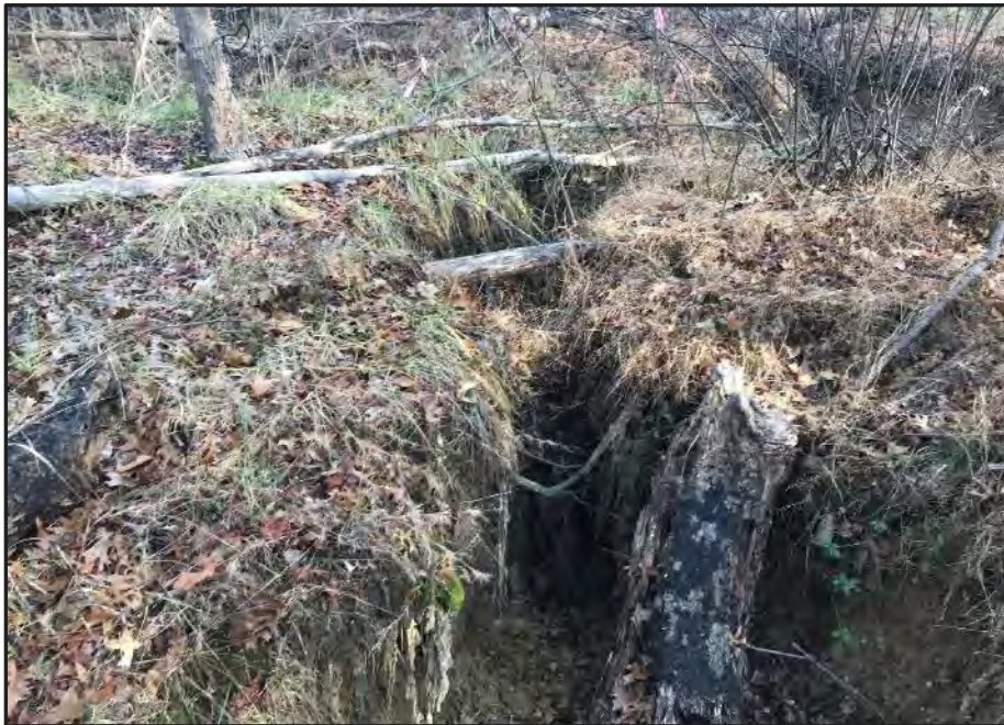
Photo 32: WUS C-16, upstream (Facing North)
