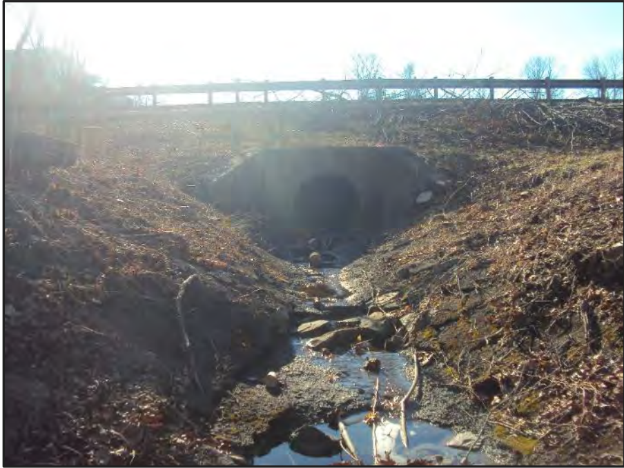
Photo 12: WUS 5D, upstream (Facing South)
