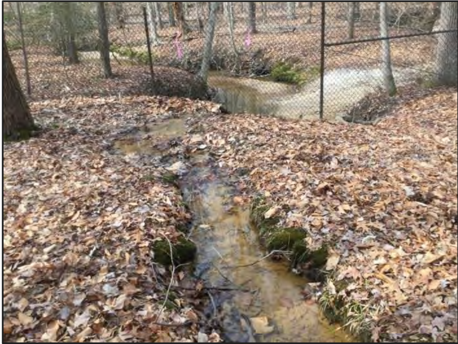
Photo 5: WUS I-3, downstream (Facing Northwest)
