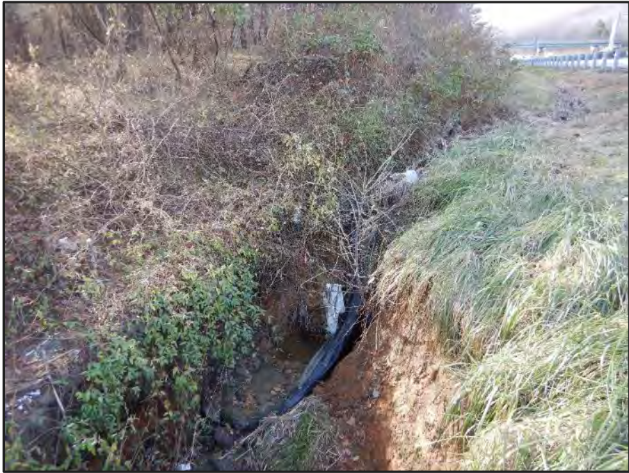
Photo 80: WUS E, upstream (Facing West)
