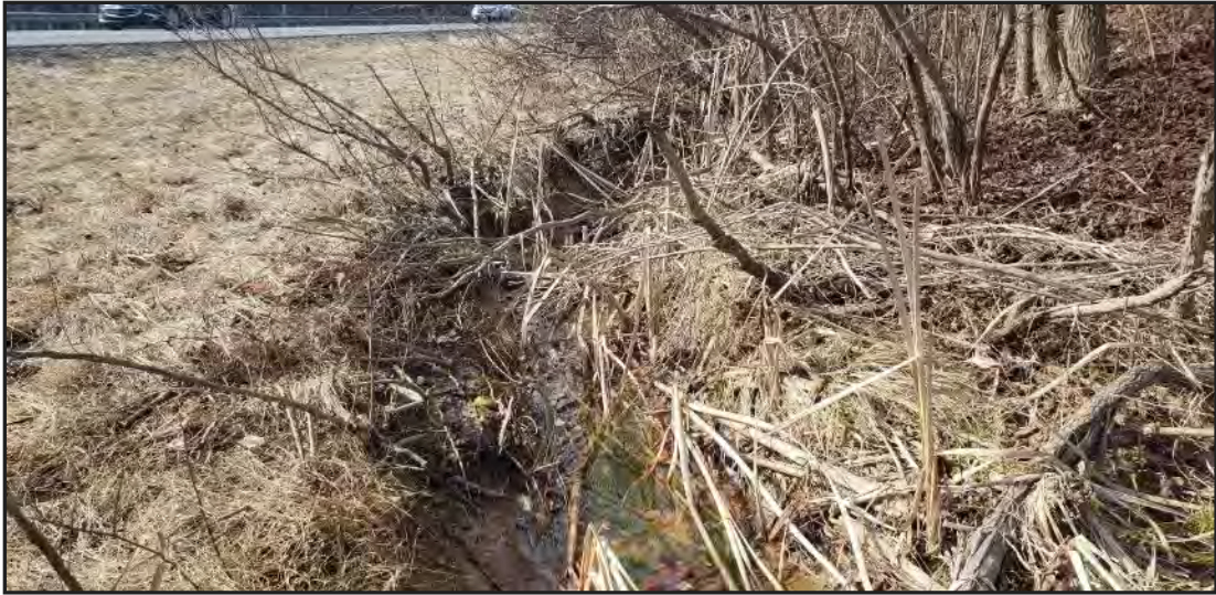
Photo 37: WUS G-20, upstream (Facing West)
