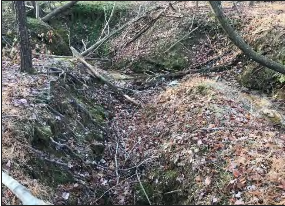
Photo 27: WUS C-14, downstream (Facing Southwest)
