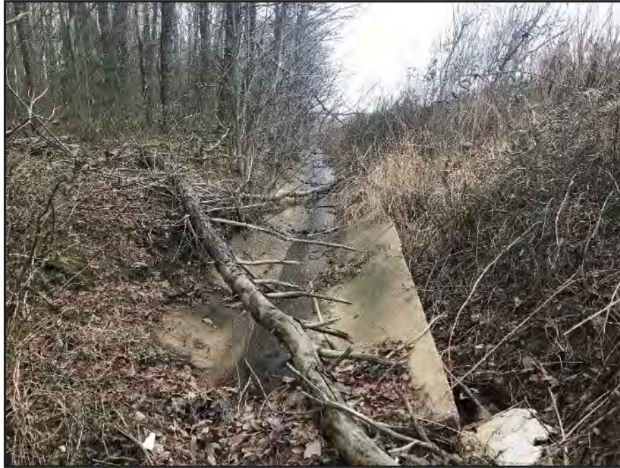
Photo 43: WUS 1D, upstream (Facing West)
