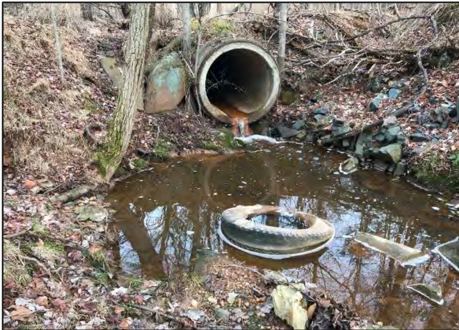
Photo 42: WUS C-21, upstream (Facing North)
