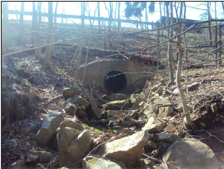
Photo 6: WUS 2D, upstream (Facing South)
