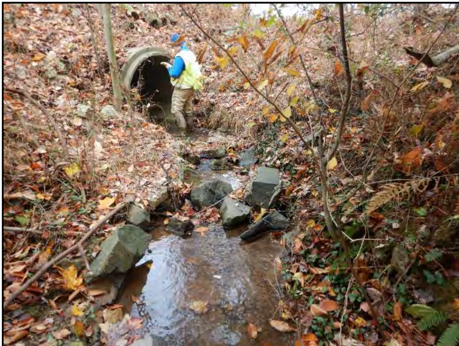
Photo 9: WUS F-1, upstream (Facing North)
