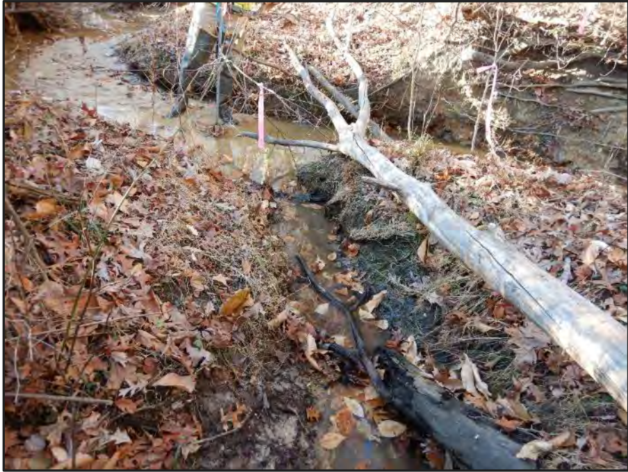
Photo 24: WUS A-12, downstream (Facing West)
