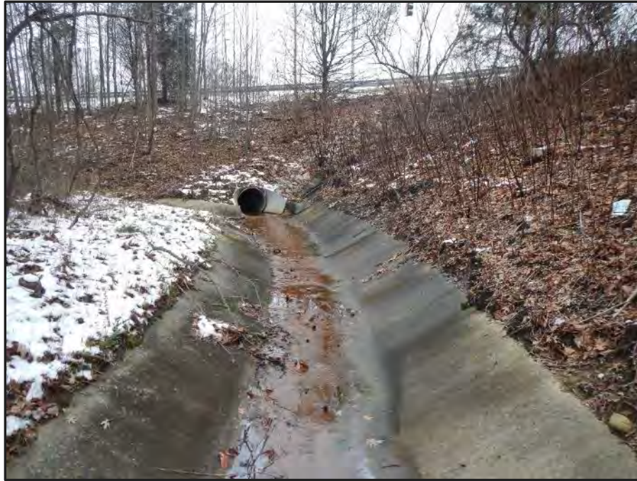
Photo 41: WUS A-21, upstream (Facing North)
