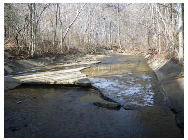
Facing upstream from Sta. 14+44 (invert of upstream end I-95 culvert) showing broken concrete lining to be removed).
