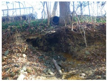
Facing left bank at severe erosion at 21" stormdrain outfall off of Randolph.
