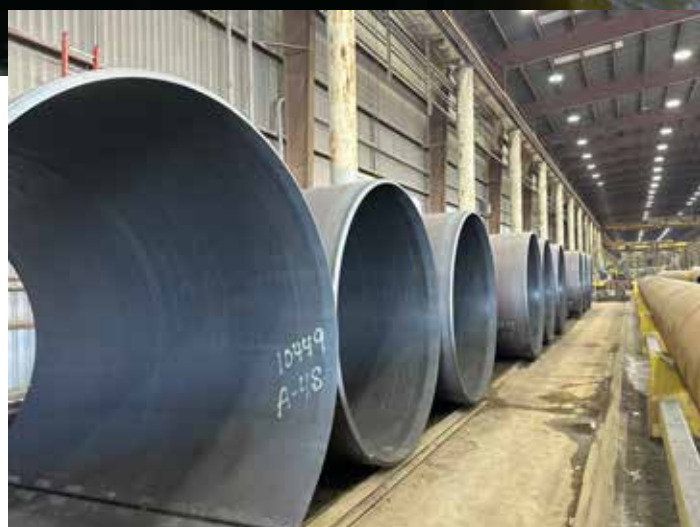
Test pile fabrication.
