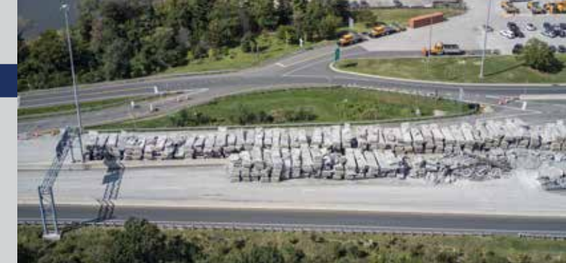
Concrete removed from former Key Bridge.
