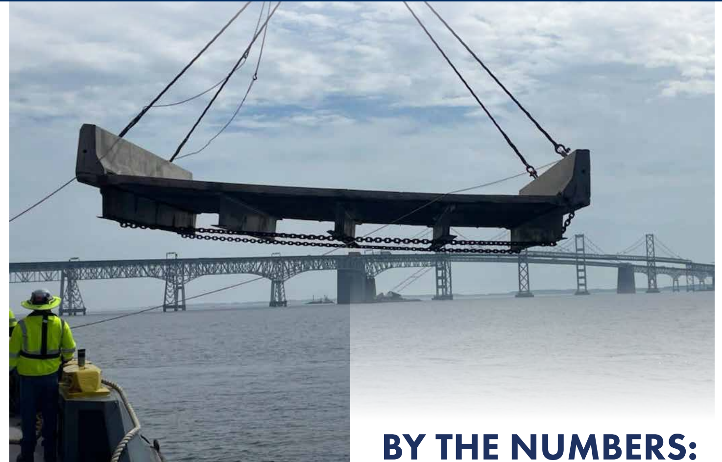
Crews moving precast deck panels into place.
