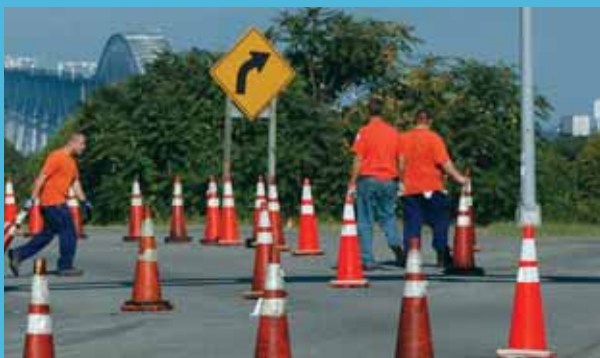
FROM TOP LEFT TO RIGHT: MARYLAND TRANSPORTATION AUTHORITY POLICE ON PATROL NEAR THE KEY BRIDGE; MARYLAND HOUSE (I-95); KAREN MOORE - SHOP ADMINISTRATIVE TECH.; POLICE SECURITY CHECKPOINT AT HATEM BRIDGE; JOE GEISLER - HEAVY EQUIPMENT MAINTENANCE TECHNICIAN; MAINTENANCE CREW AT THE BAY BRIDGE.
