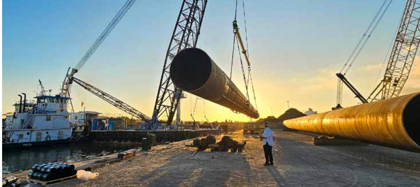
Key Bridge Rebuild, Test Pile Delivery
