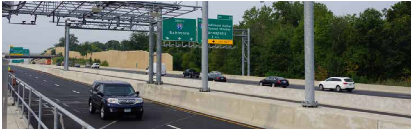
I-95 Express Toll Lanes
