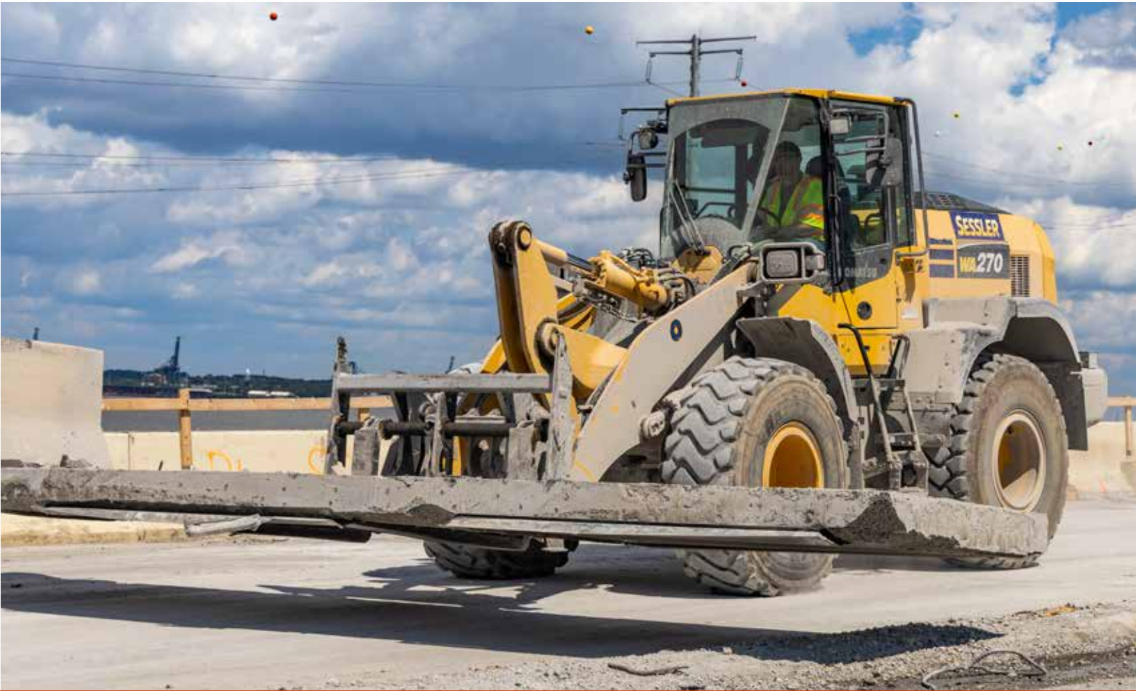
Key Bridge Rebuild Mechanical Demo
