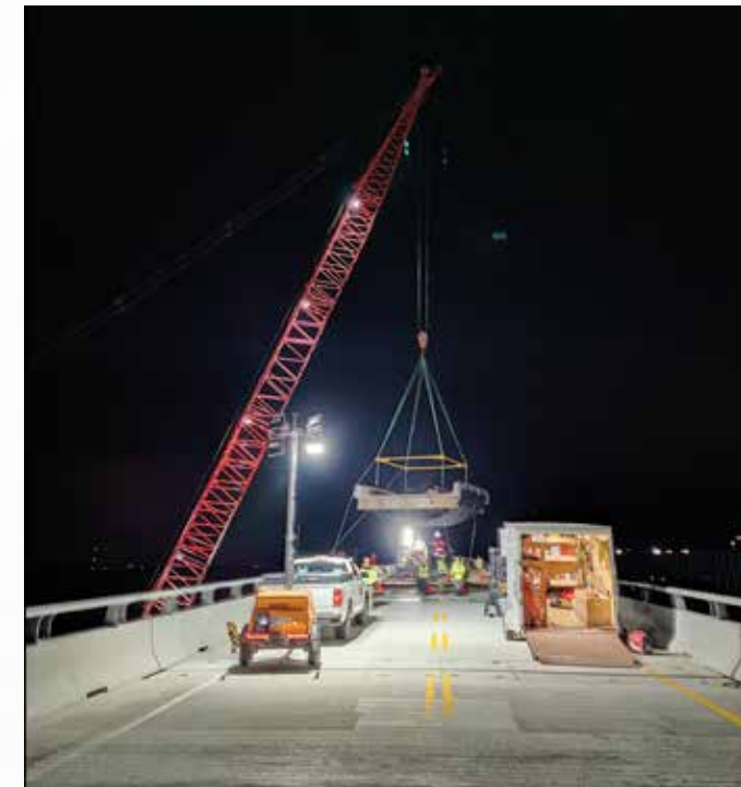
Bay Bridge Eastbound Deck Replacement – March 2025
