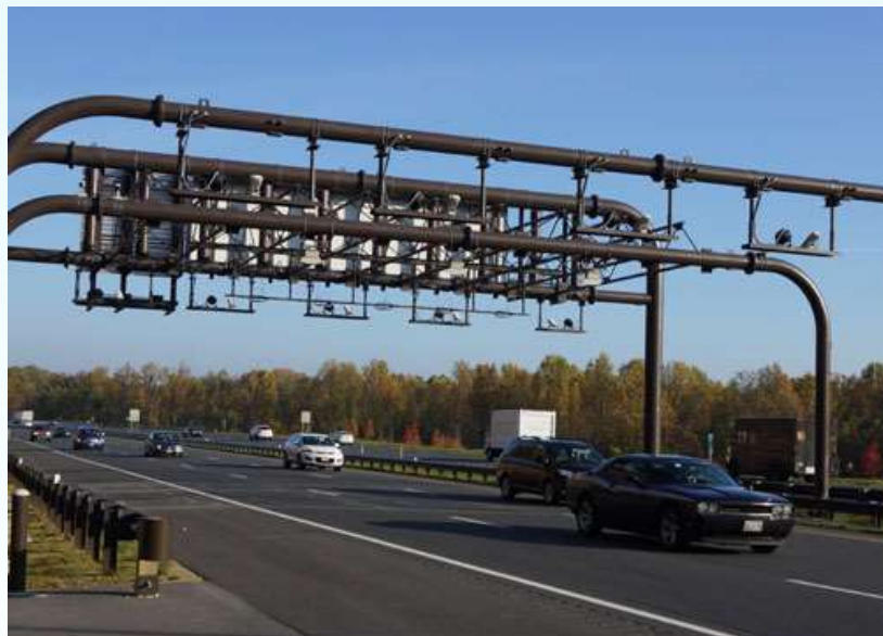
Figure 5: Sample Gantry Along the ICC / MD 200
