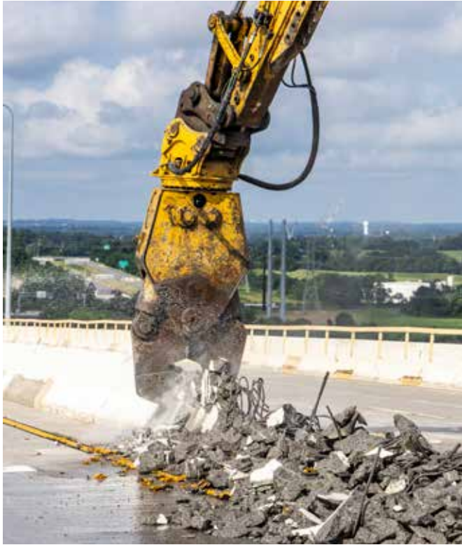
Key Bridge Demolition - Deck Removal
