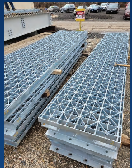
Temporary joint grates.
