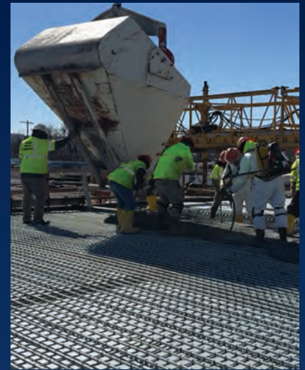
Crews working on pre-cast decks.
