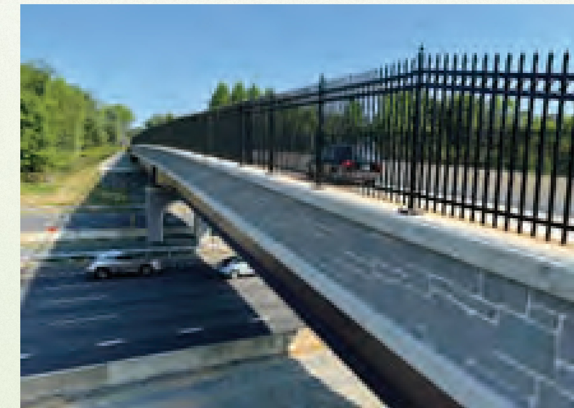
Replaces 50 year old bridges
