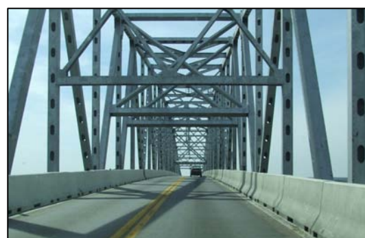
Photo V-2: Nice Bridge from travel lanes
