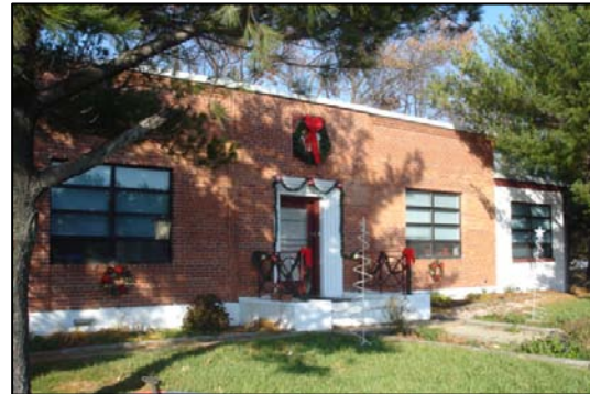
Photo V-3: Potomac River Bridge Administration Building
