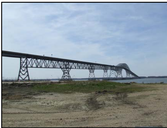
Photo III-1: View of Nice Bridge from Aqua-Land Marina and Campground, in Charles County, Maryland, looking southwest.
