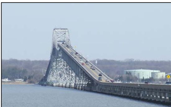
Photo V-1: Nice Bridge from the Virginia shore
