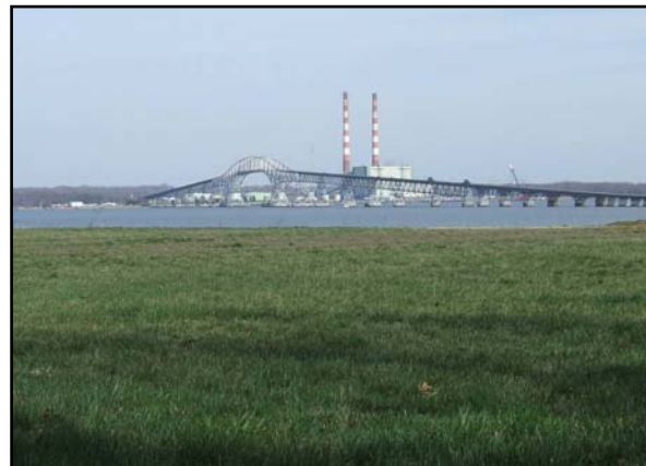
Photo III-2: View of Nice Bridge from Roseland Road, in King George County, Virginia, looking southeast with the Morgantown Generating Station in the background.
