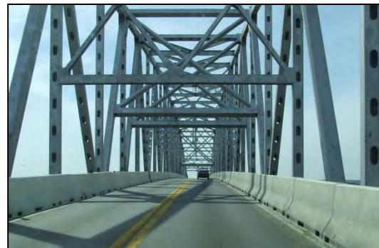
Photo 2: Nice Bridge from travel lanes
