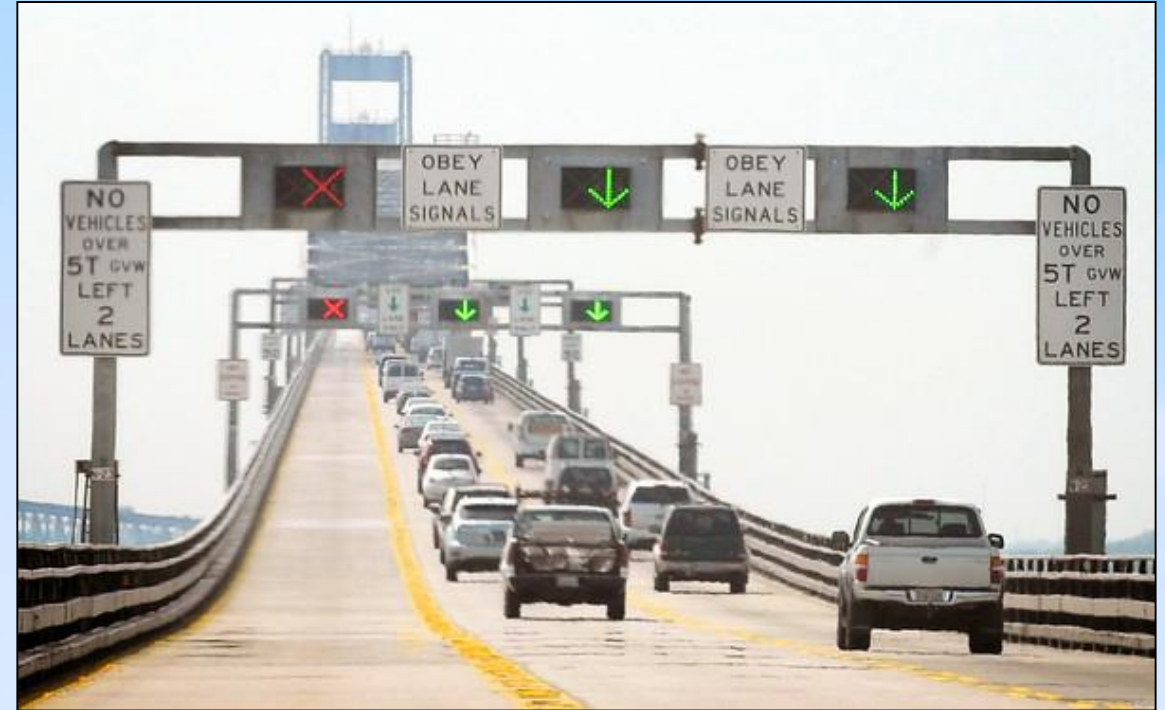
Bay Bridge lane-use control signals
