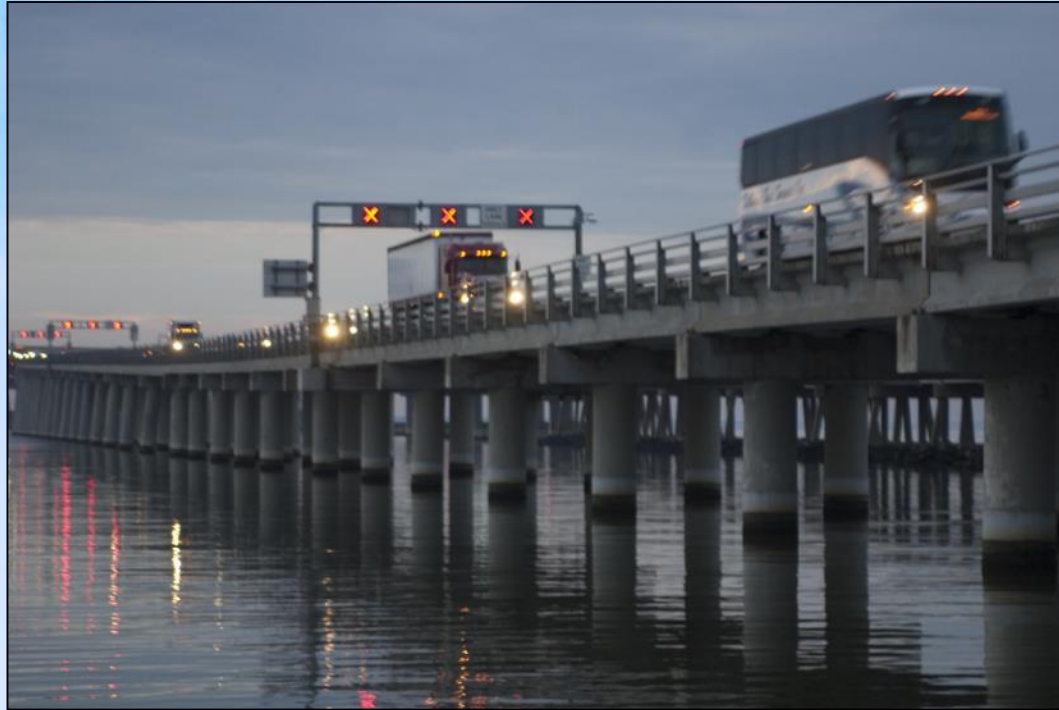
Bay Bridge lane-use control signals
