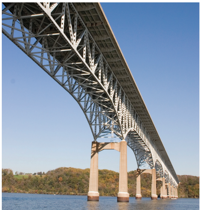
The Tydings Bridge on I-95
