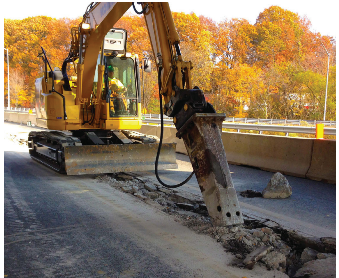
Superstructure Replacement on I-895 over Patapsco Flats
