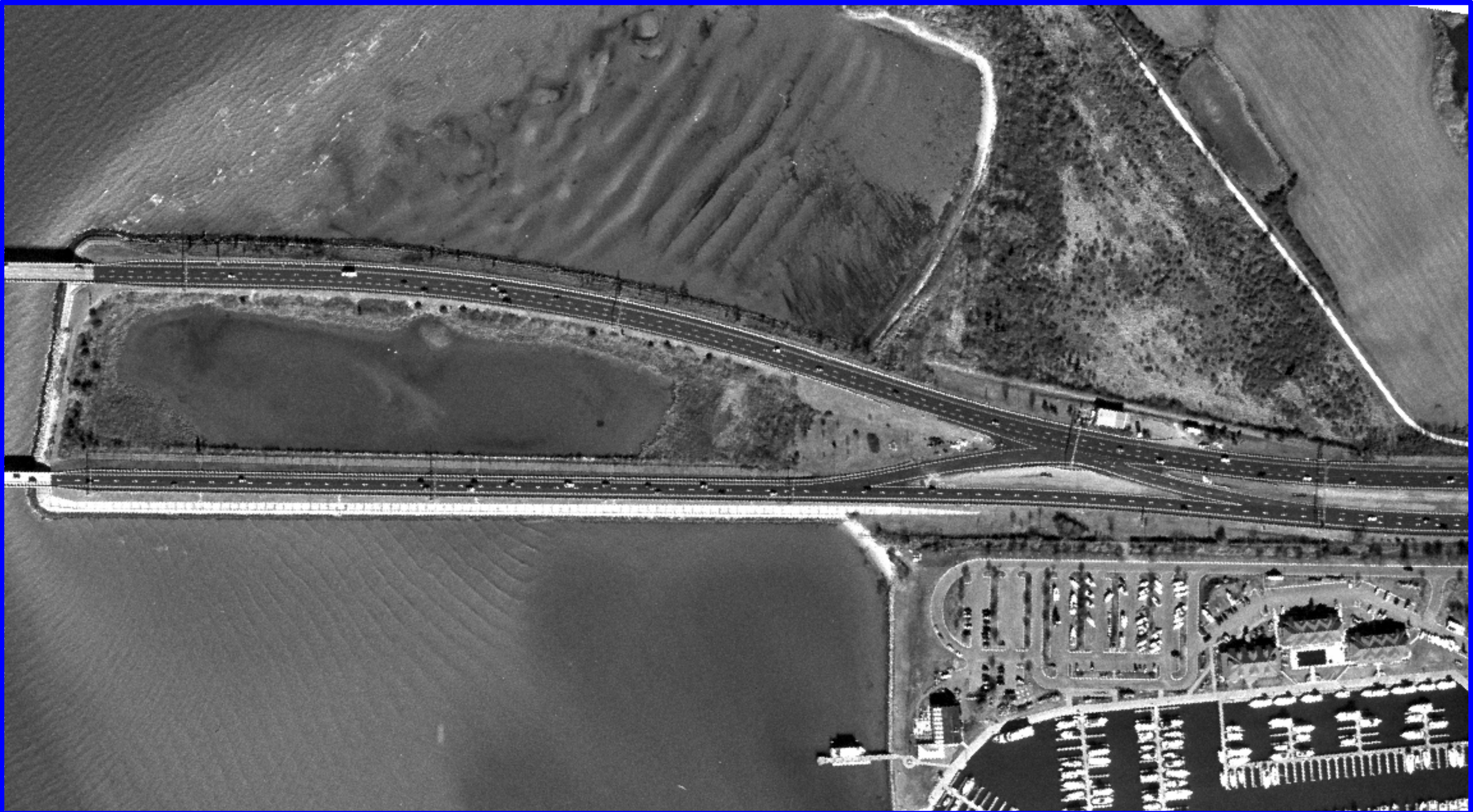
FIGURE C-2 BAY BRIDGE (EAST APPROACH)
