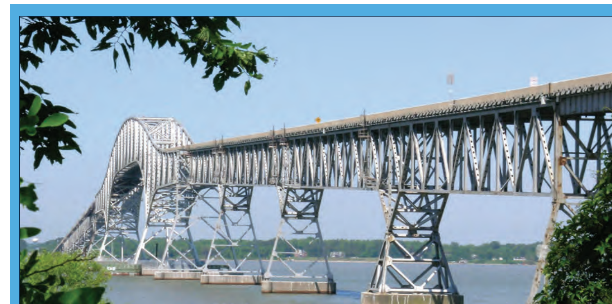
Harry W. Nice Memorial Bridge
