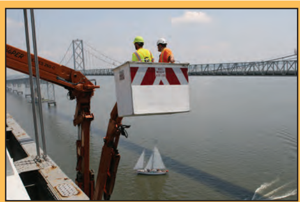
Bridge inspection at the Bay Bridge
