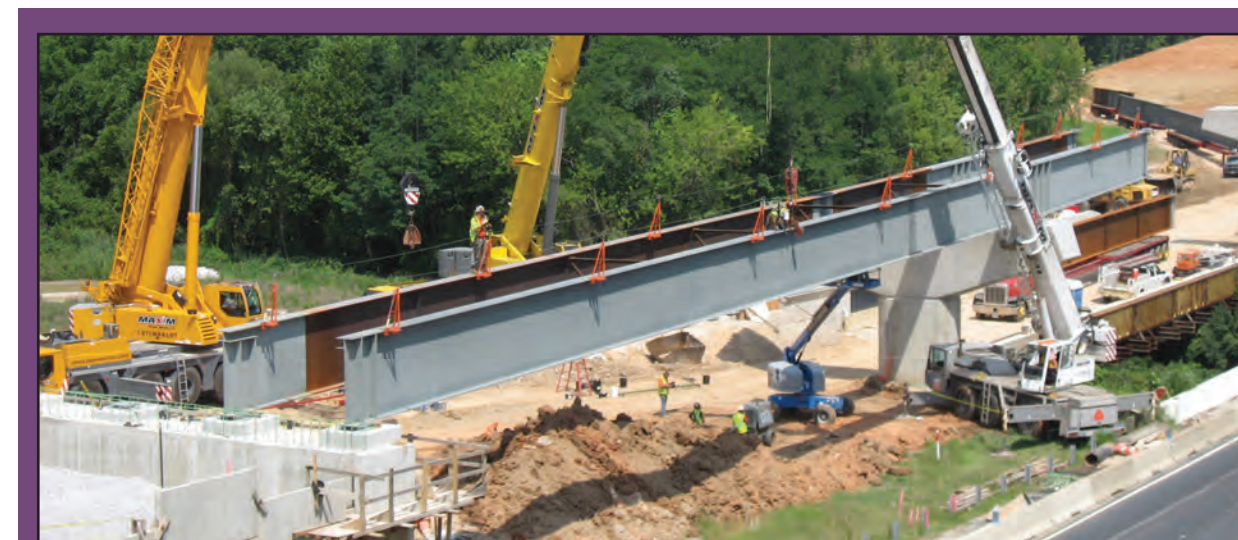
Steel setting for I-95/I-895 interchange
