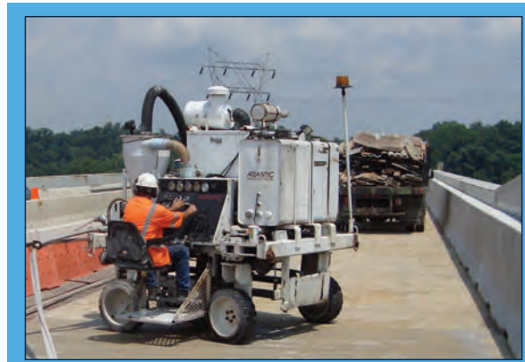
Hatem Bridge deck rehabilitation
