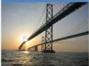
Bay Bridge (US 50/301)
