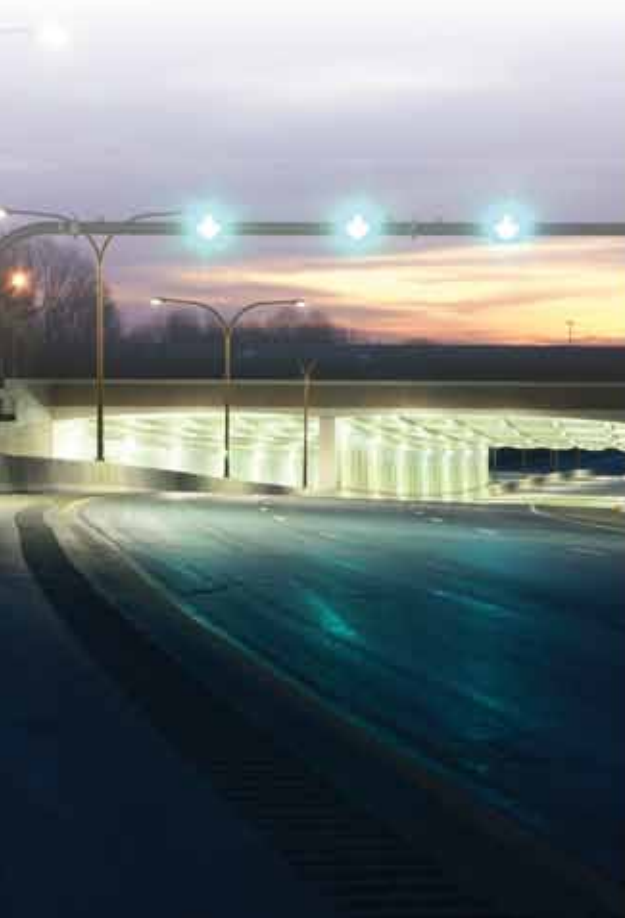
Intercounty Connector Deckover in Montgomery County
