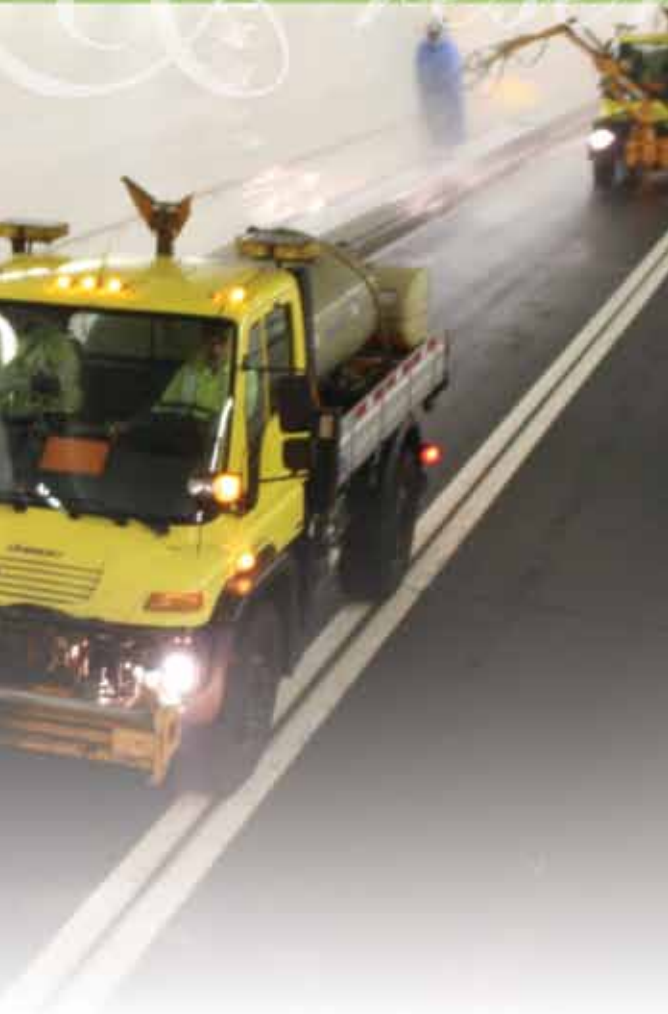
Unimog washing the walls of the Fort McHenry Tunnel
