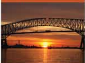
Francis Scott Key Bridge (I-695)
