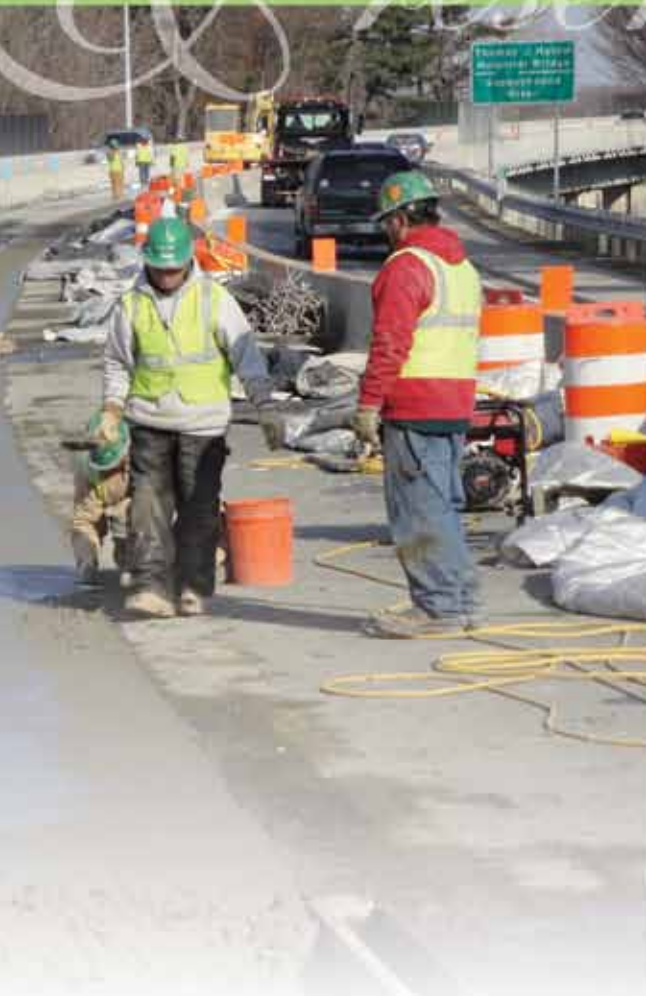
Re-decking the Thomas J. Hatem Memorial Bridge
