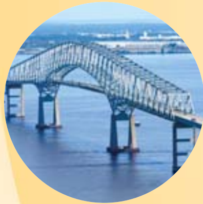
Francis Scott Key Bridge (I-695)
