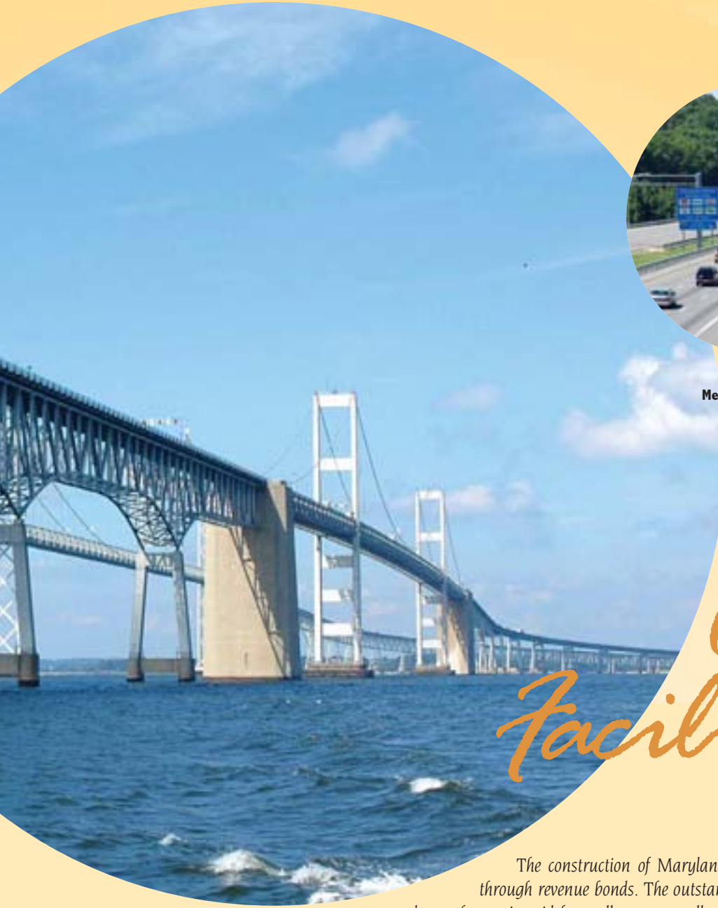
William Preston Lane Jr. Memorial (Bay) Bridge (US 50/301)
