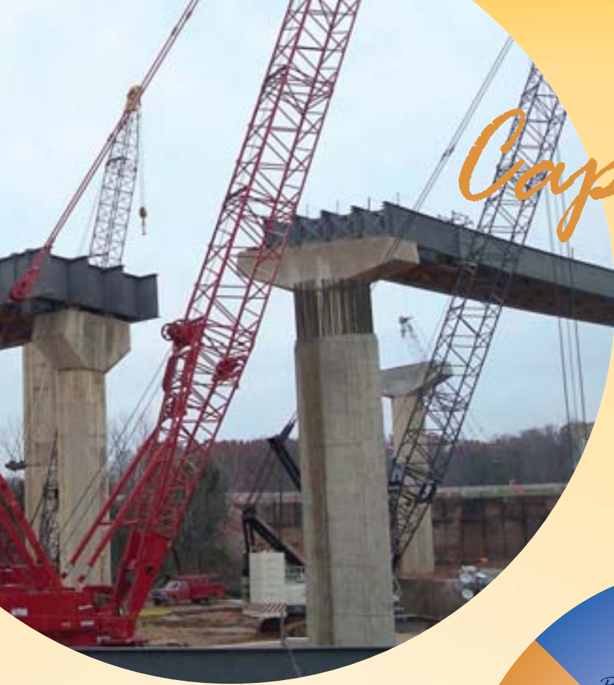
I-95/I-695 interchange construction as part of the ETLs SM project.
