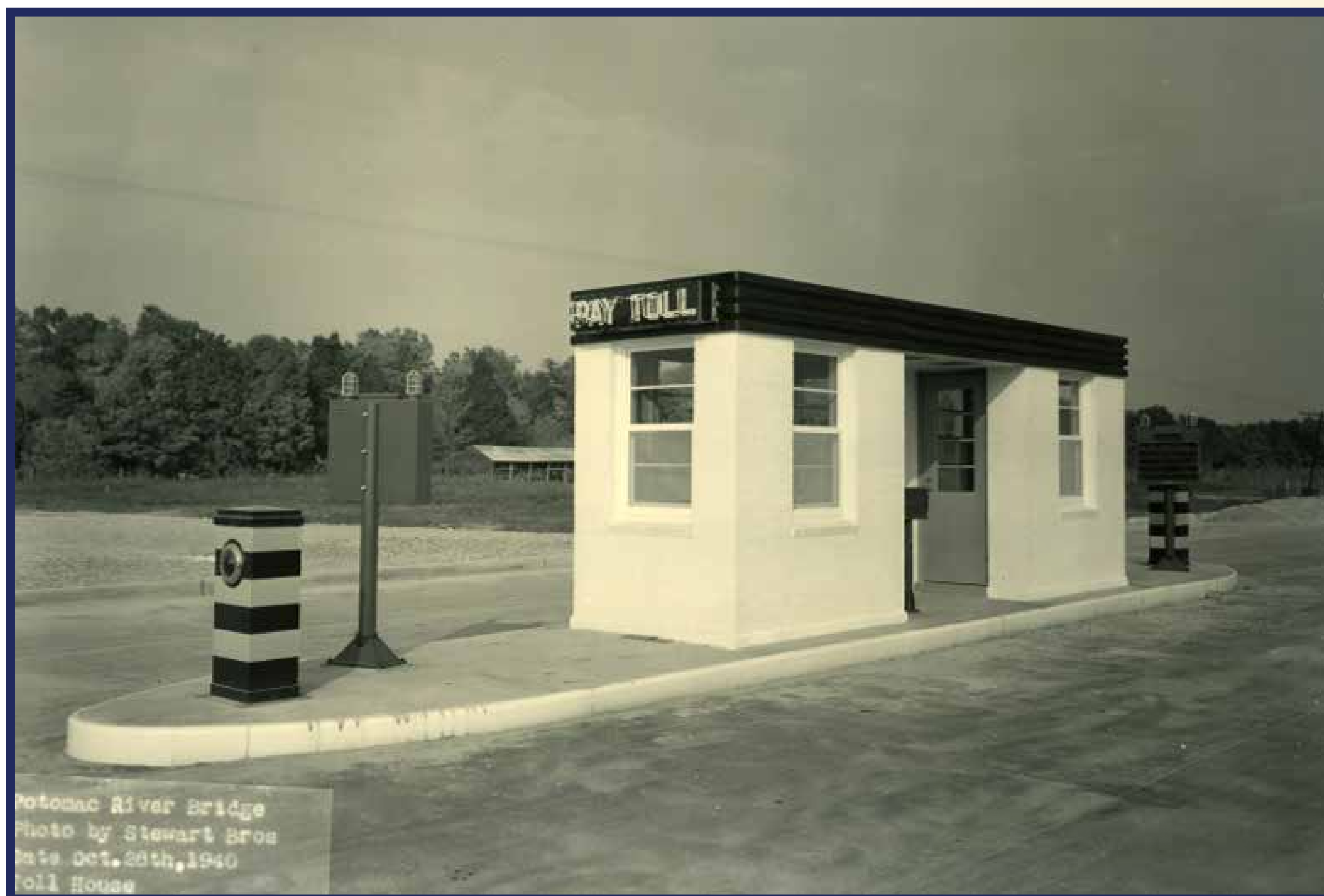
Original Maryland toll plaza, 1940
