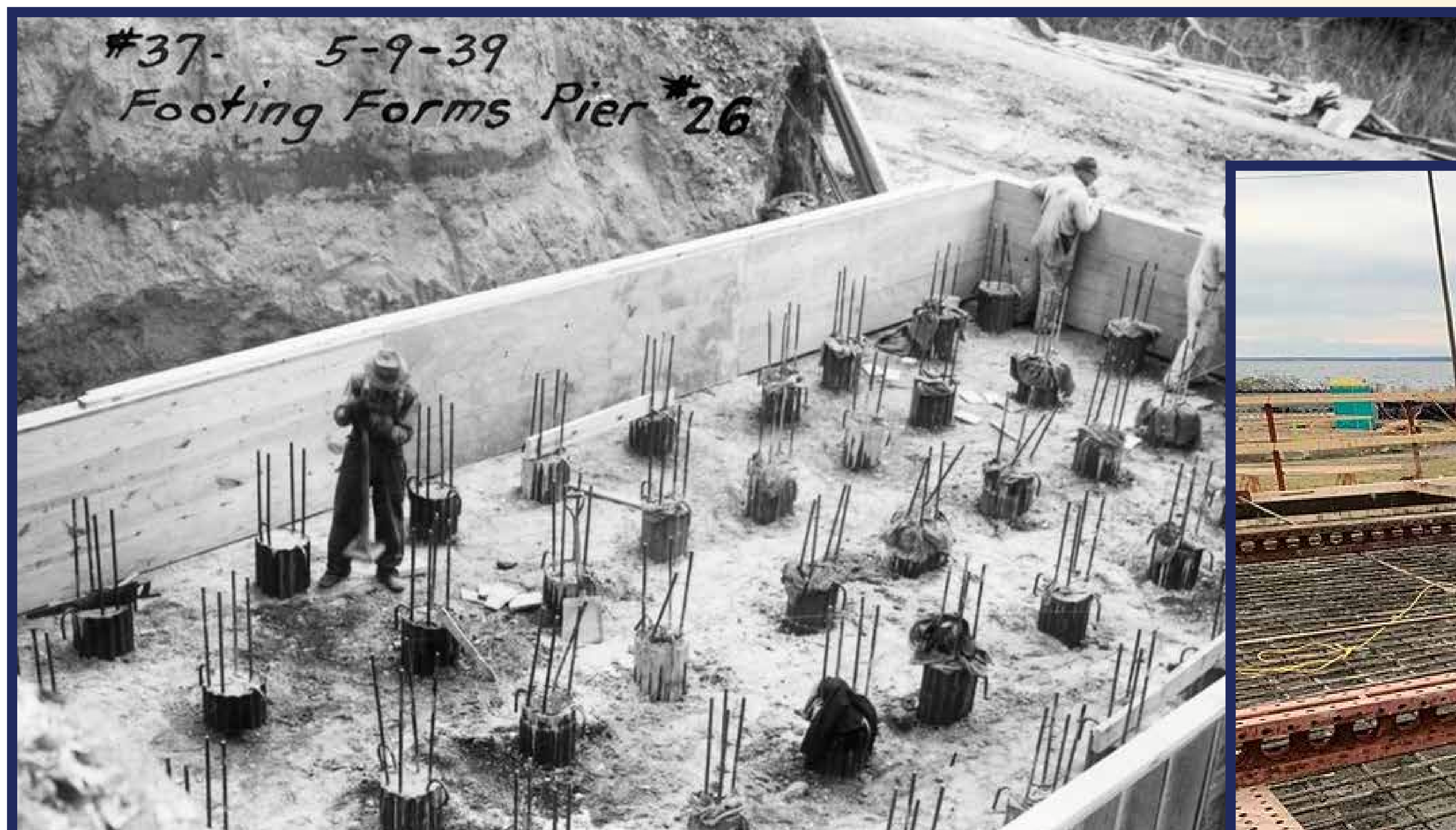
Pier concrete footings, 1939
