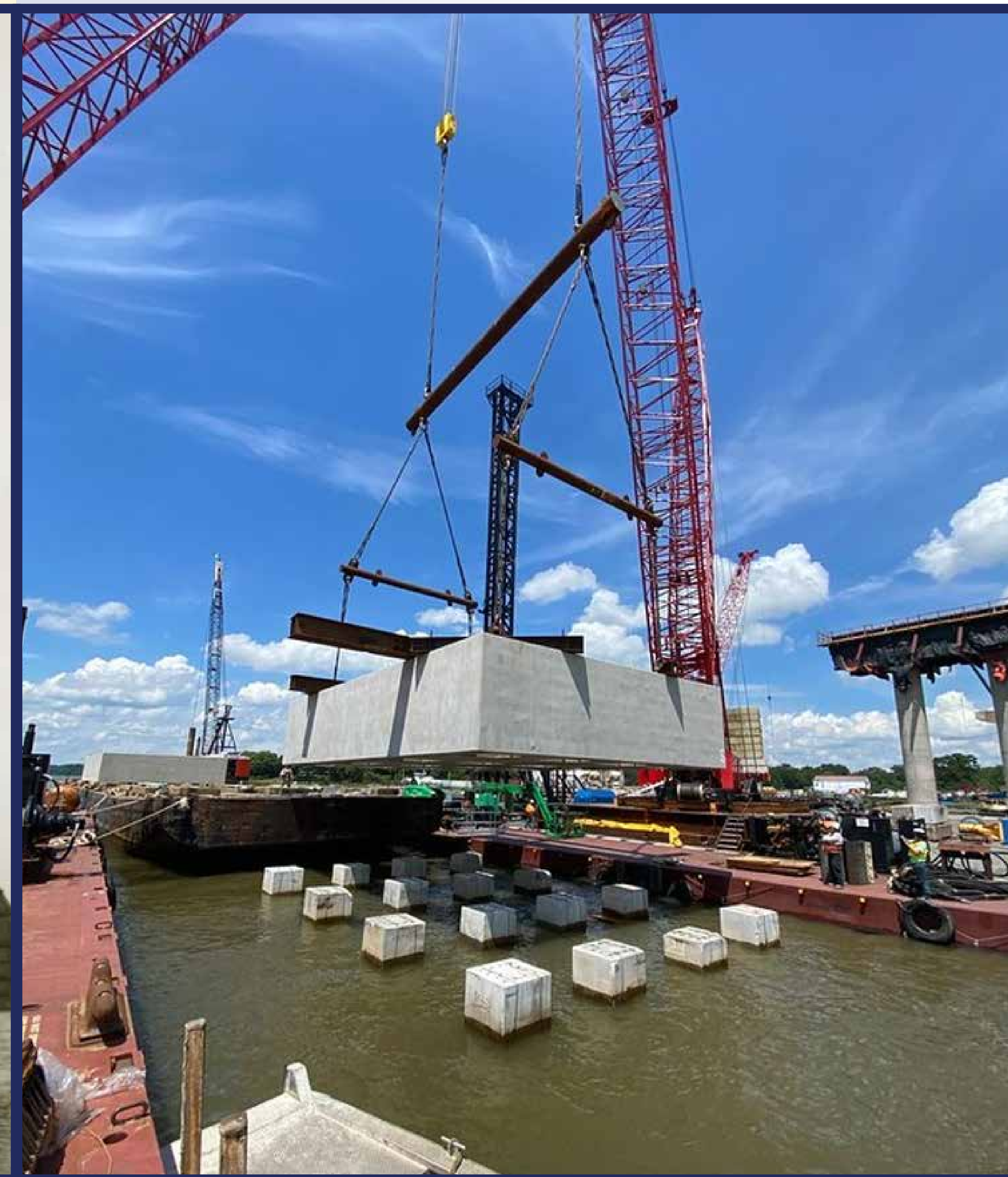
Form and footing placements, 2021
