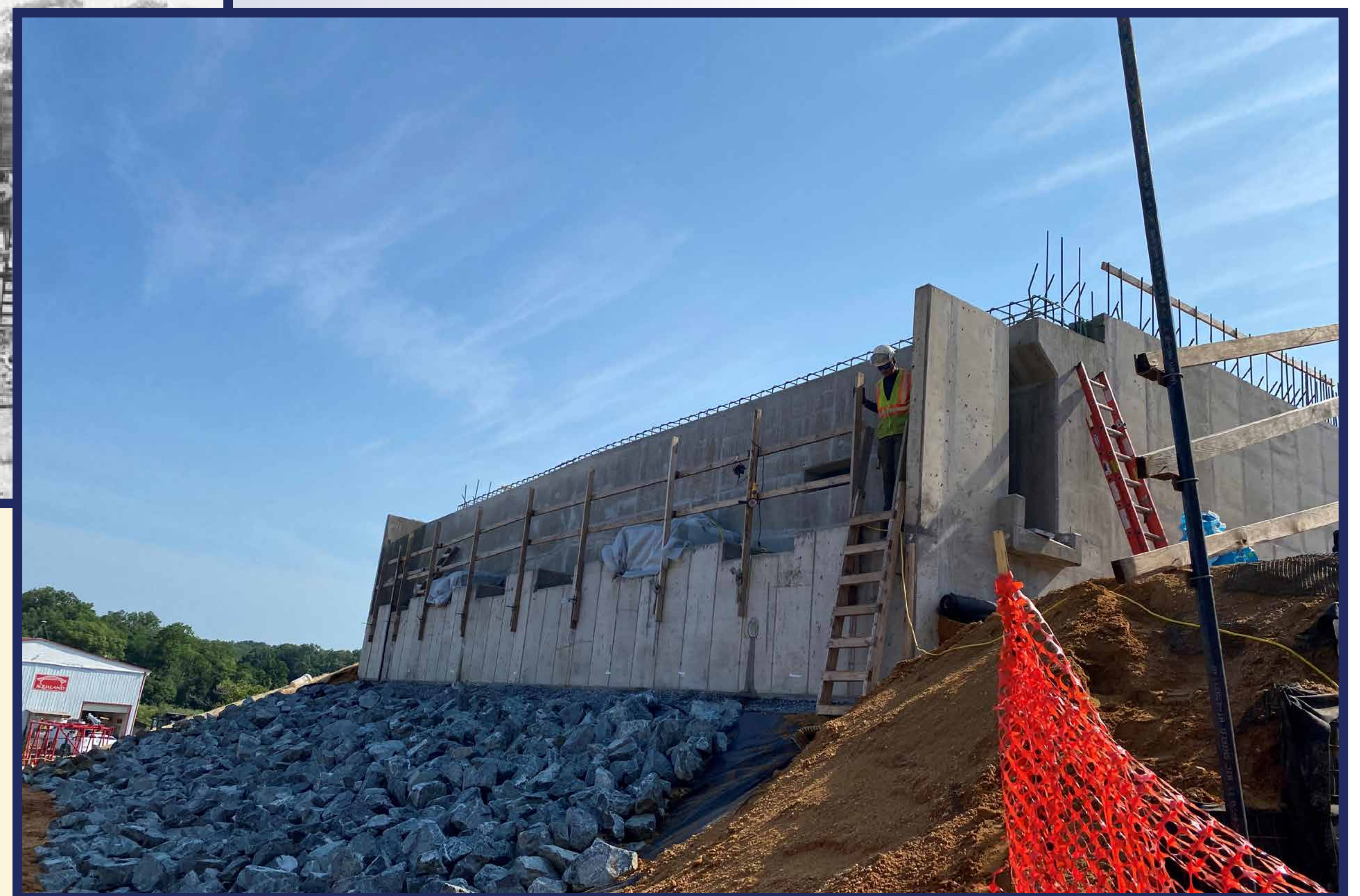
Maryland bridge abutment work, 2021
