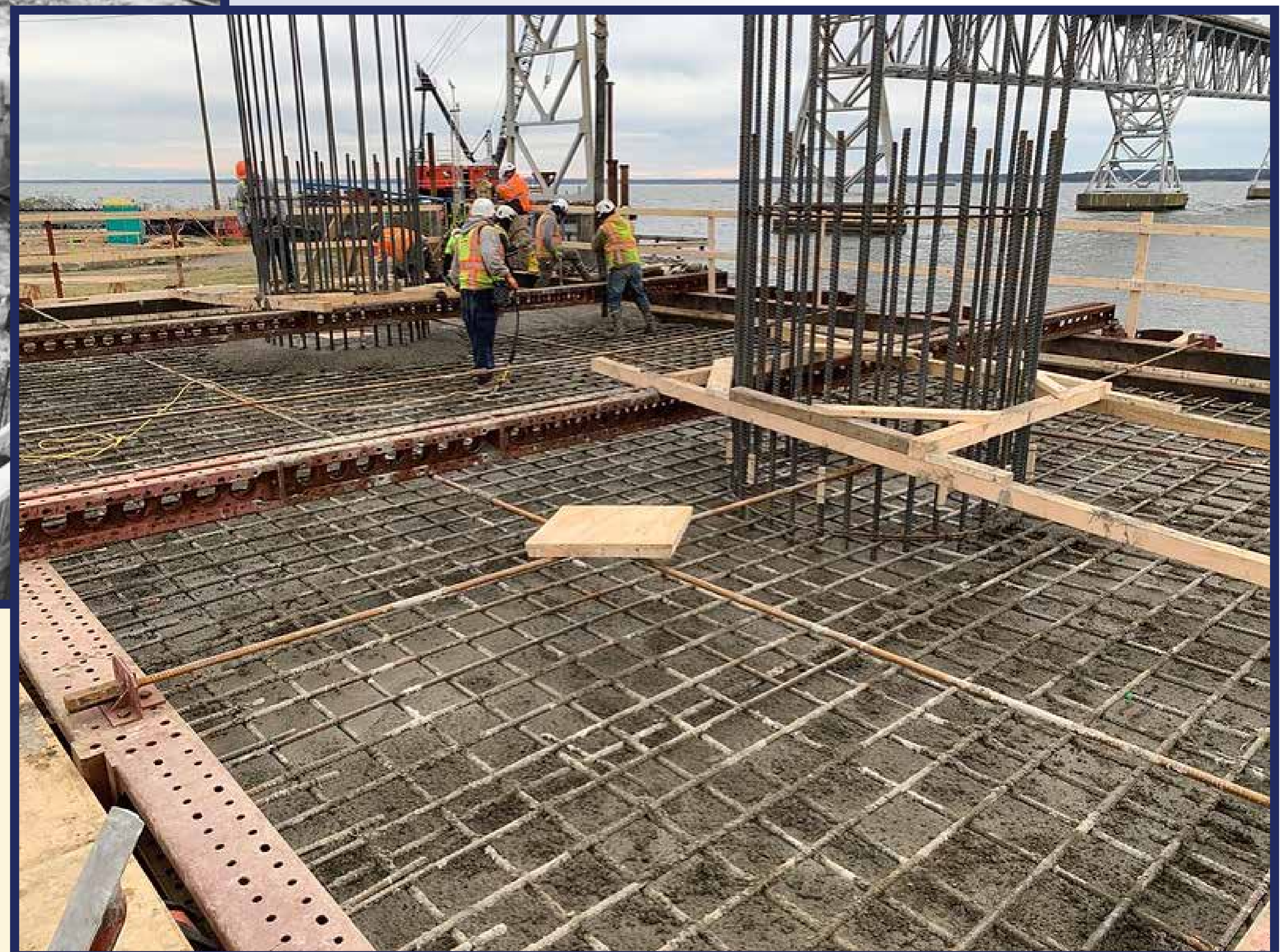
Pier concrete footings, 2021
