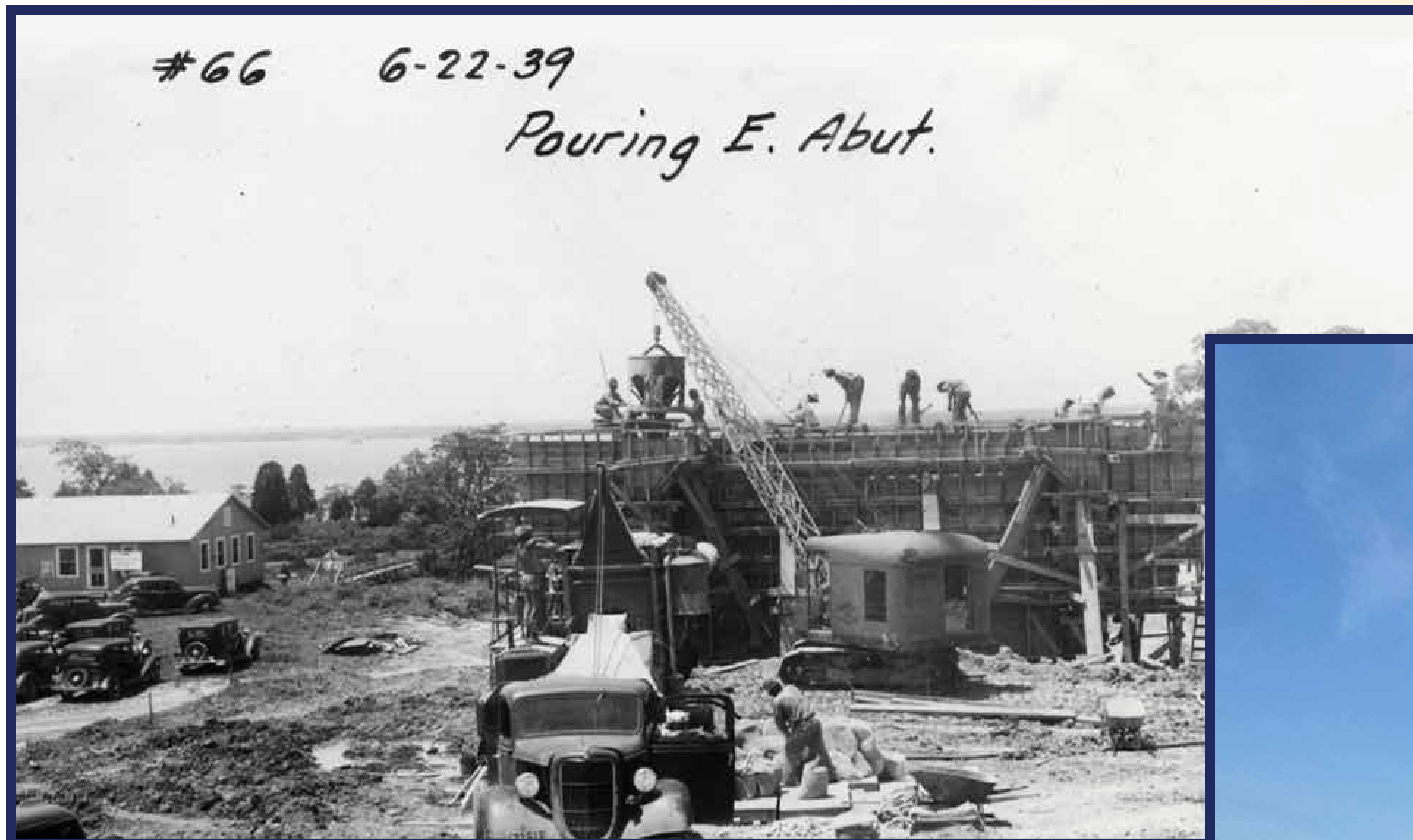
Maryland bridge abutment work, 1939
