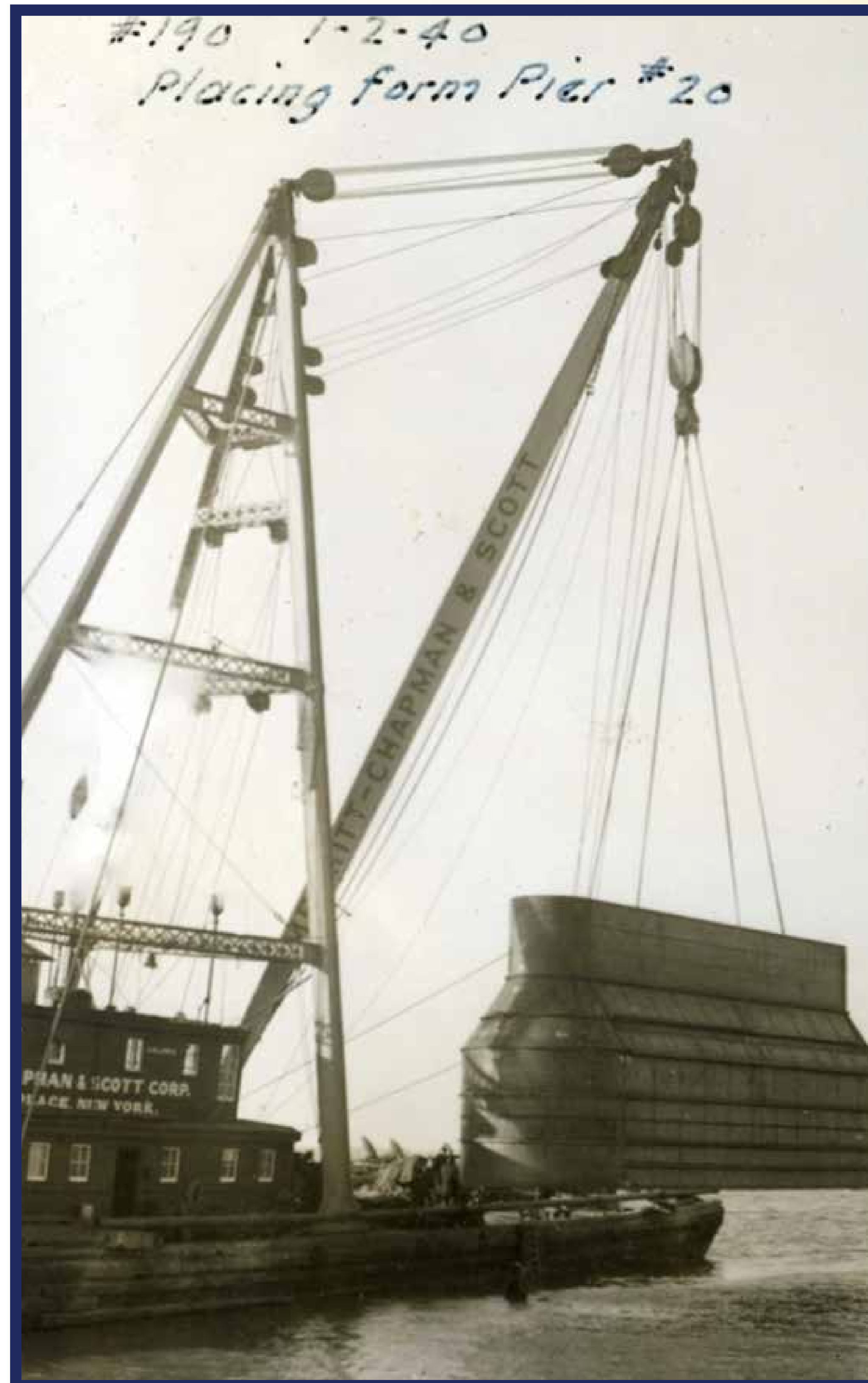
Form and footing placements, 1940
